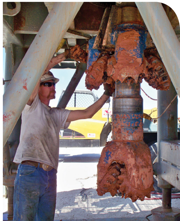
Construction of a TWDB-funded water supply project on the Colorado River
