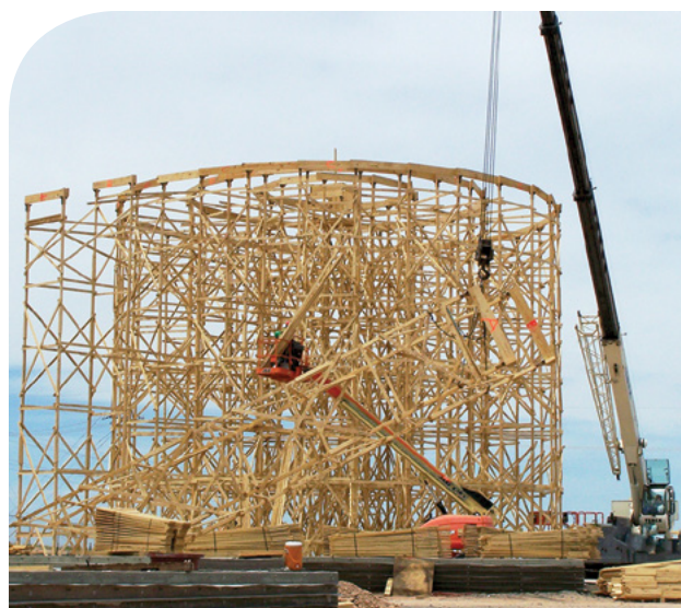
Construction of a TWDB-funded ground storage tank, Amarillo, Texas
