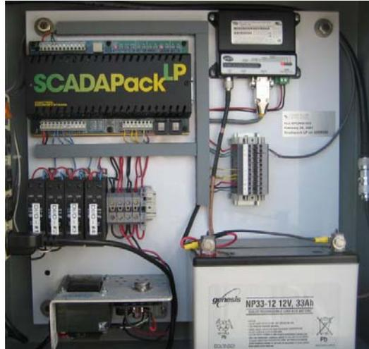
Figure 2 – Typical Telemetry Site Equipment
