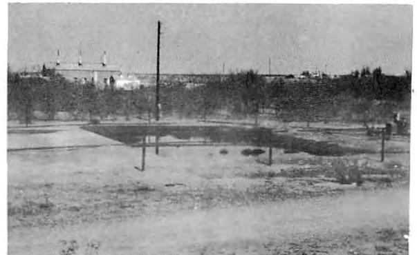
Figure 10. -- Brine-collection pits at Texaco Pipeline Station, NE $\frac{1}{4}$ , NW $\frac{1}{4}$  Section 33, Block 32, T-3-N, T & P RR Survey, Howard County. Pit on left is asbestos-cement lined to prevent seepage. Brine is pumped from pits to disposal well. View is east.
