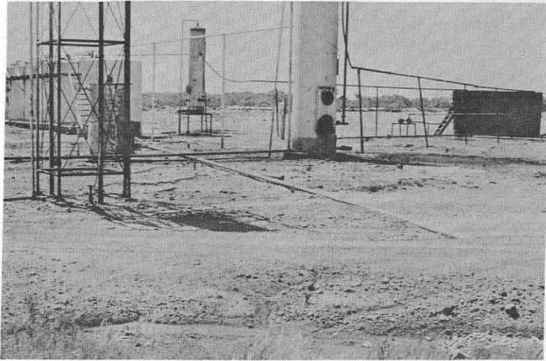
G. Tank battery with oil-salt water treaters and salt water storage tank, NE $\frac{1}{4}$  Section 163, BBB & C RR Co. Survey (Area 1, Figure 11). View is west.
