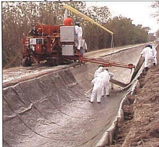
Mobile equipment is used to produce and install the polyurethane fabric lining on site. Installers are trained on the safe handling and use of the material, including what to do in case of a spill.
