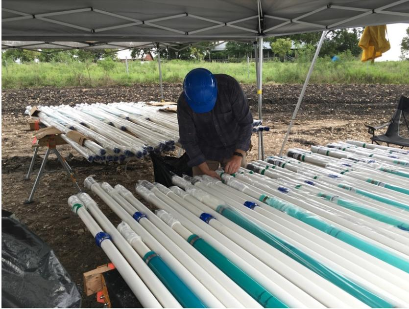
**Figure C-3. Layout of Westbay equipment prior to installation of the multiport well.**
