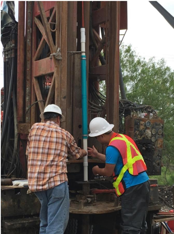
**Figure C-4. Multiport well apparatus installation.**
