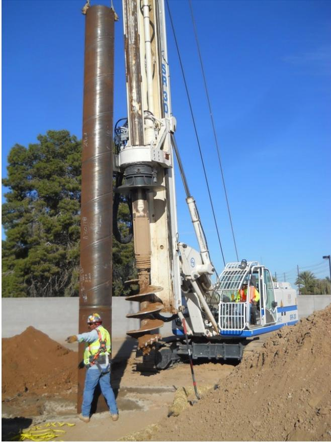
**Figure D-1. Lowering the surface casing into the borehole.**
