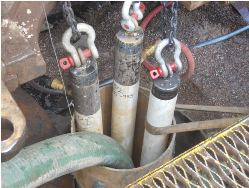
**Figure D-2. Installation of the three individual nested piezometers for the Deer Valley nested well.**
