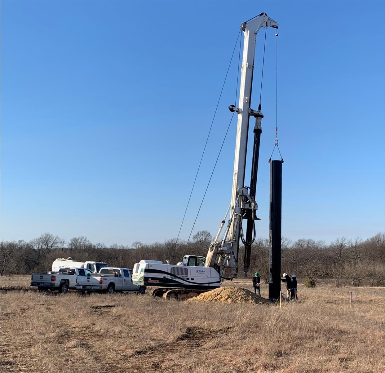
**Figure 3-13. Installing conductor casing.**
