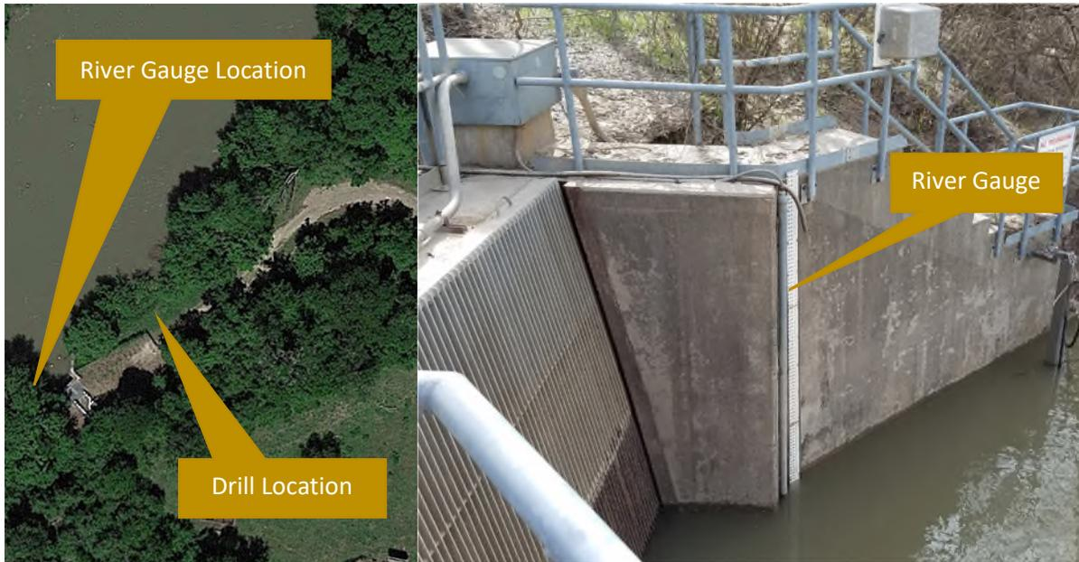
Aerial view of Study Site No. 1: Sam Gideon Power Plant Intake Facility, showing the river gauge and drill locations (left) and an image showing the river gauge (right).
