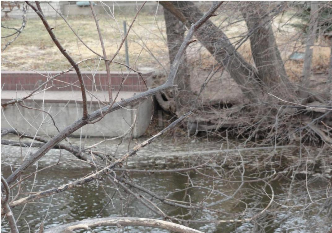
Figure 8. Bank failure due to undercutting and overland erosion.
