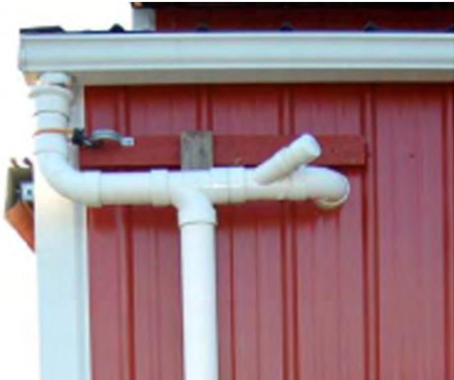
Roof gutter, Y valve connector and downspout on barn, Larrison residence, Georgetown
