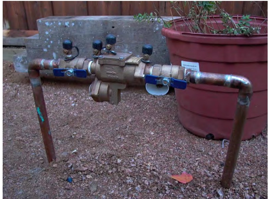
Backflow prevention device, McMahan residence, Dallas, Texas
