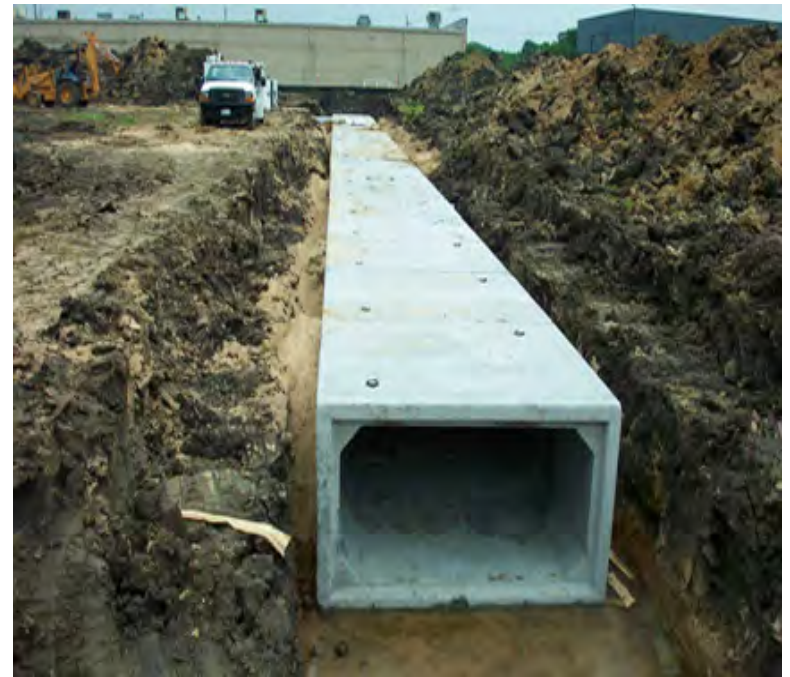
Concrete culverts (Medical Center, Webster, Texas)
