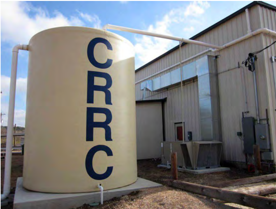
Fiberglass tank, Community Resource and Recreation Center, Canyon Lake, Texas
