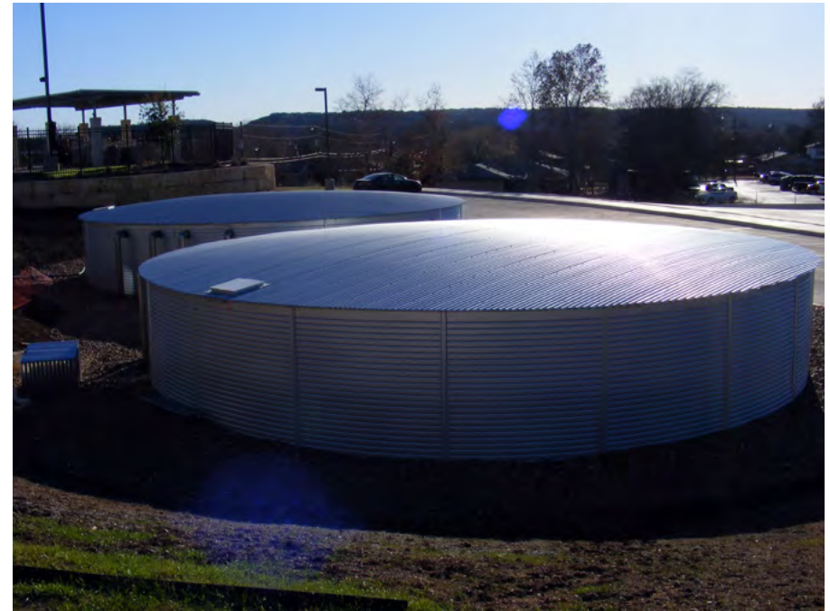
Galvanized metal tank with food-grade liner, Salvation Army Recreation Center, Kerrville, Texas
