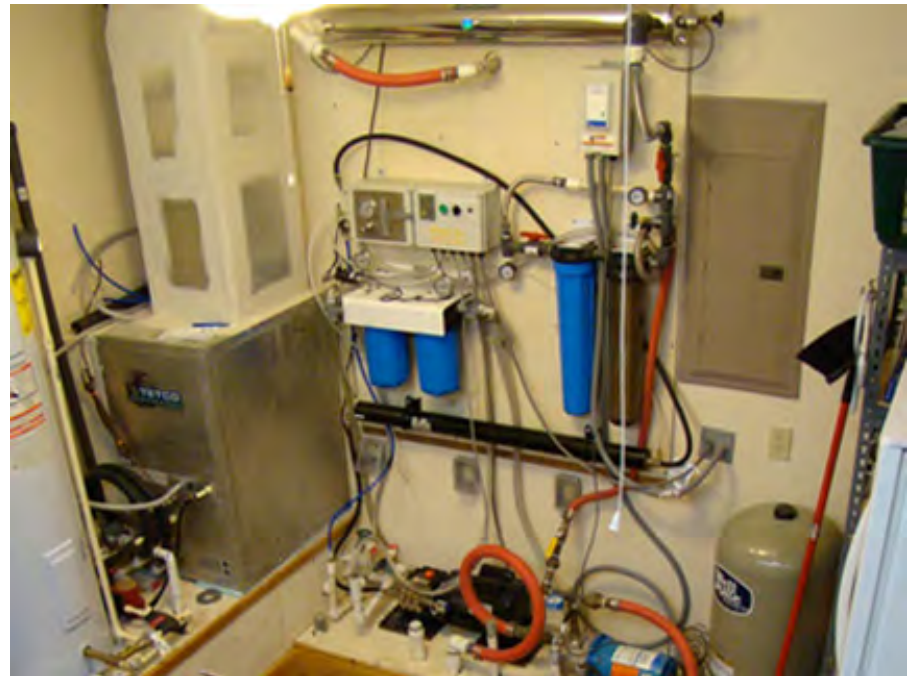
Sediment and sand filters, UV lamp, and pumps, Moore residence, Taft, Texas
