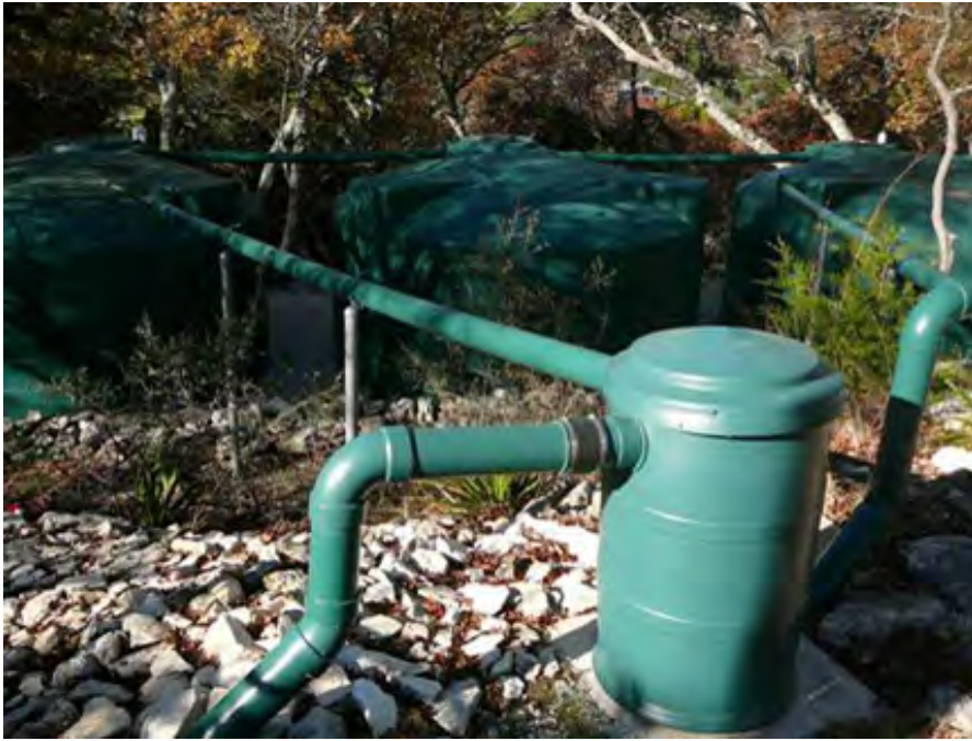
First-flush washer with sock filter, Kight residence, Boerne
