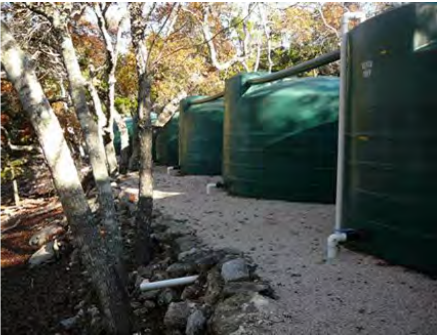
Polyethylene tanks (Kight residence, Boerne, Texas)
