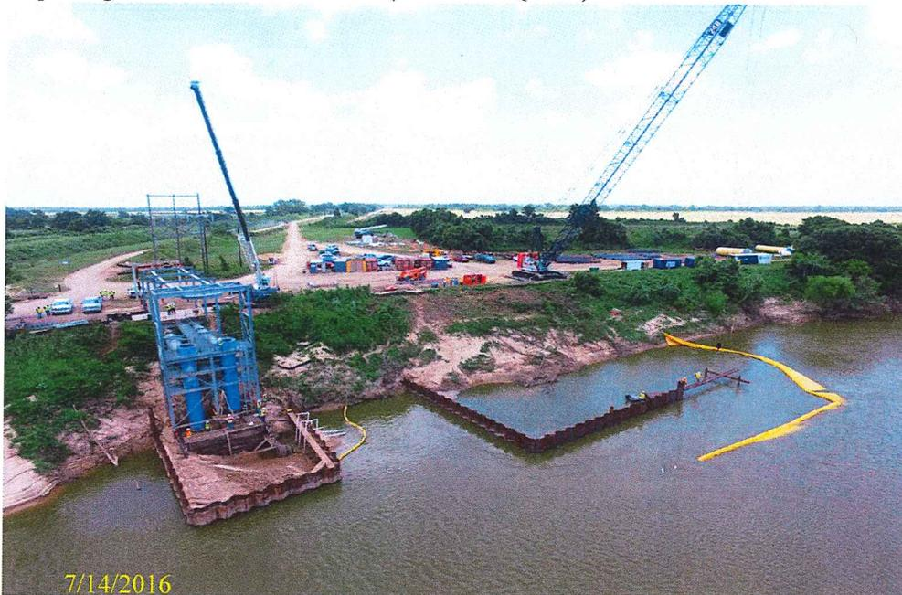
Figure 3 - Riverside View of Temporary Cofferd Dam for River Outfall
