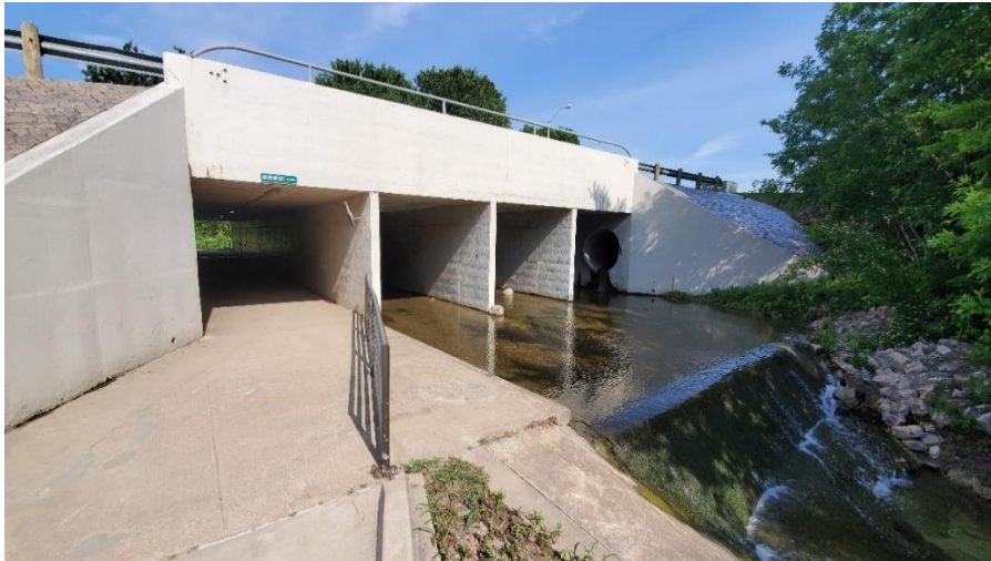
Figure 2.40 Staged or Tiered Culvert Design used in North Texas with Multiple Culvert Sizes and Flow Elevations
