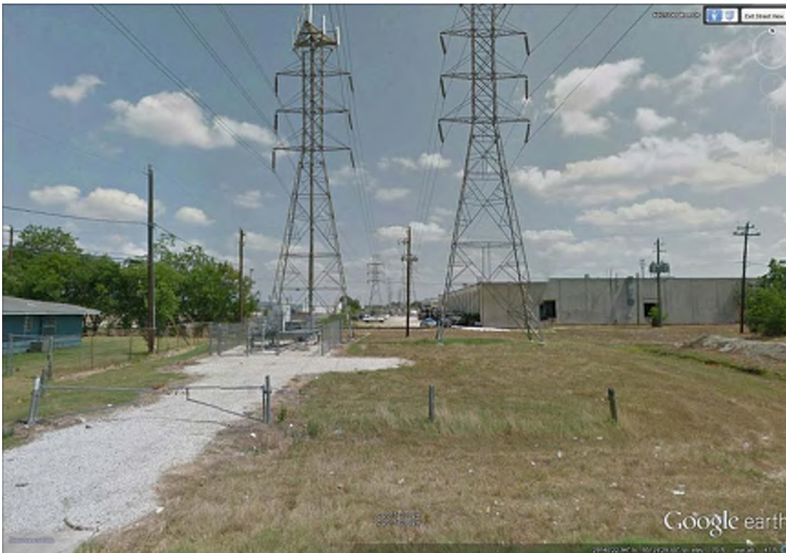
Figure 5: Transmission Towers and Electric Sub-Station Located at Doulton Drive
