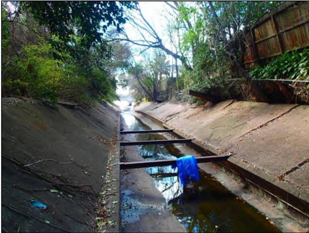
Figure 2-6: View of Temporary Stabilization Measures Along Project Reach (2015)
