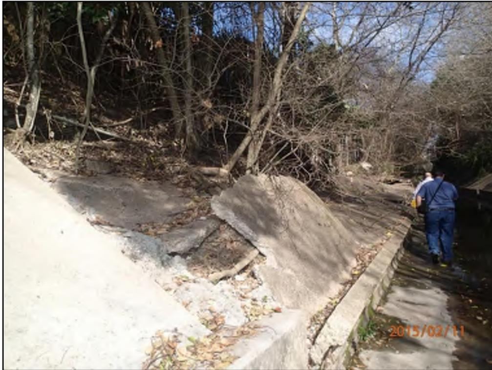
**Figure 2-4: View of Concrete Buckling Damage Along Project Reach**
