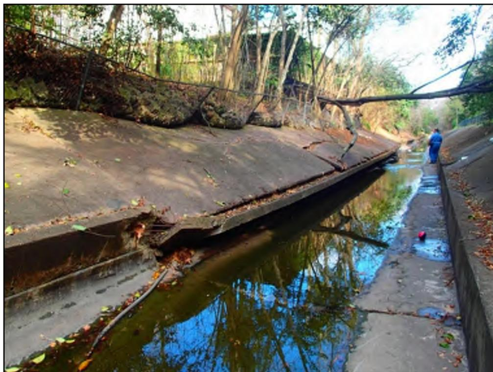
**Figure 2-5: View of Concrete Pavement Damages Along Project Reach**
