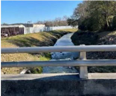
Figure 2-2: Halls Bayou looking upstream from Hardy Toll Road bridge
