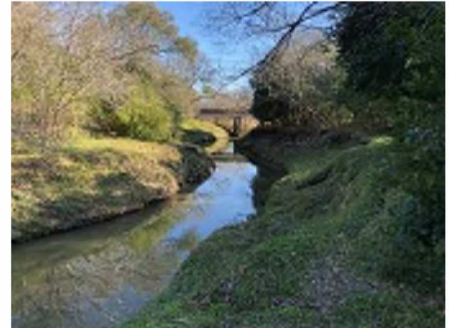
Figure 2-3: Halls Bayou looking downstream toward Hardy Toll Road bridge
