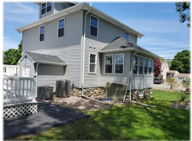
Photo of north and west side of building
