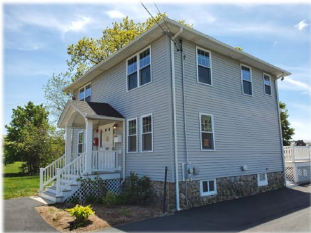
Photo of south and east side of building
