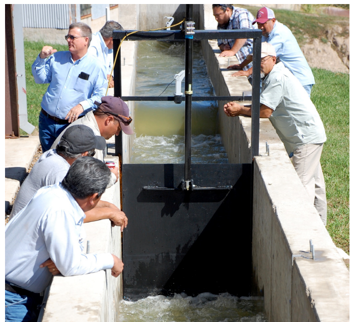
Above: Water level sensor Below: Training in auto-gate operations at the Rio Grande Center for Ag Water Efficiency
