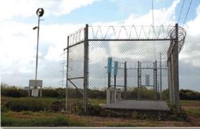
**Wind generator used to power auto gate and related SCADA electronics at the Theime Road check.**
