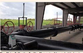
**Flow Meter Calibration Facility: Mag meter (blue and white box in the foreground) and control valves for the meter testing manifold.**
