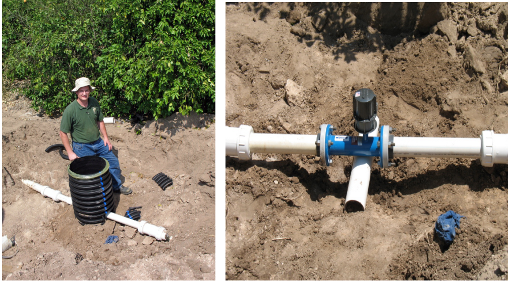
Above: Dr. Shad Nelson, Texas A&M University-Kingsville poses with 3” installation. Below: Harlingen Irrigation District technician, Richard Keating, and Eddie Esquivel of TAMUK install Siemens transit time meter.
