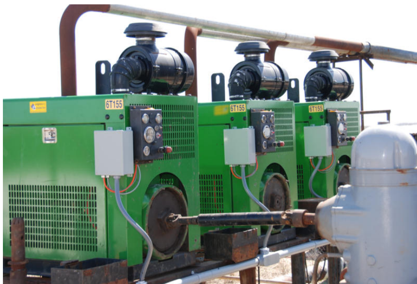
Figure 9 – Delta lake Irrigation District – Variable Speed Pumps
