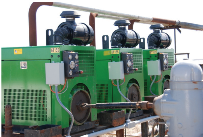
Variable speed controller components installed on the pumps and in the vandal box
