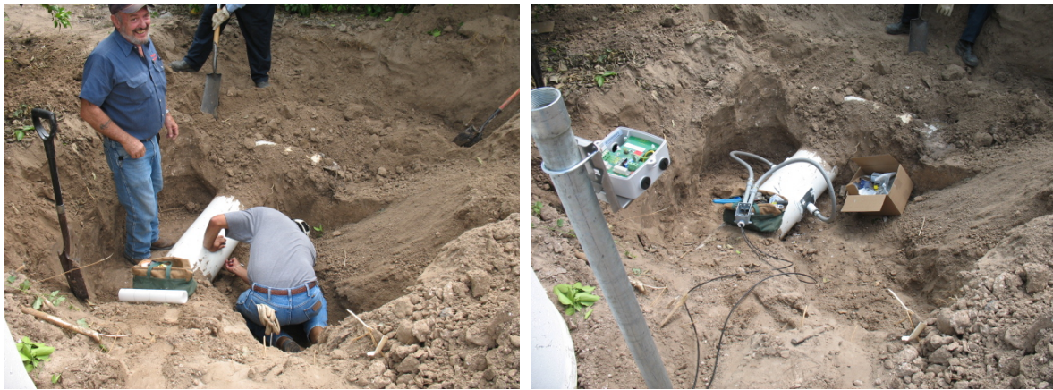
Above: Dr. Shad Nelson, Texas A&M University-Kingsville poses with 3” installation. Below: Harlingen Irrigation District technician, Richard Keating, and Eddie Esquivel of TAMUK install Siemens transit time meter.
