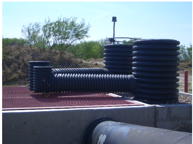
Catch Basins and Installed Flow Meter
