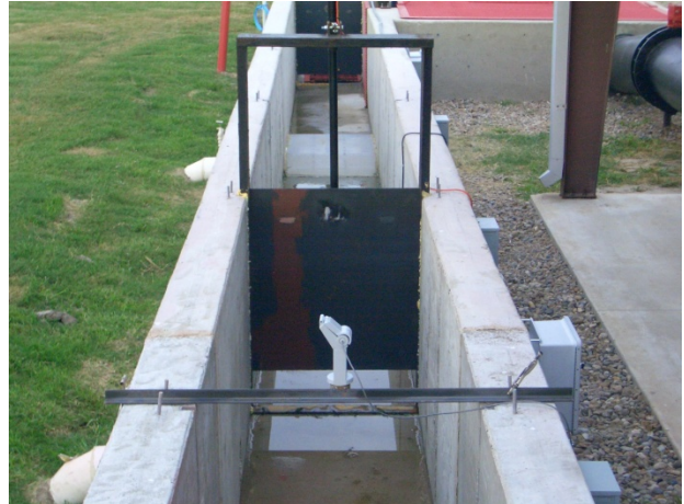
Auto Gate and Acoustic Level Transmitter
