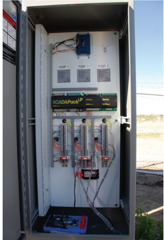
Variable speed controller components installed on the pumps and in the vandal box
