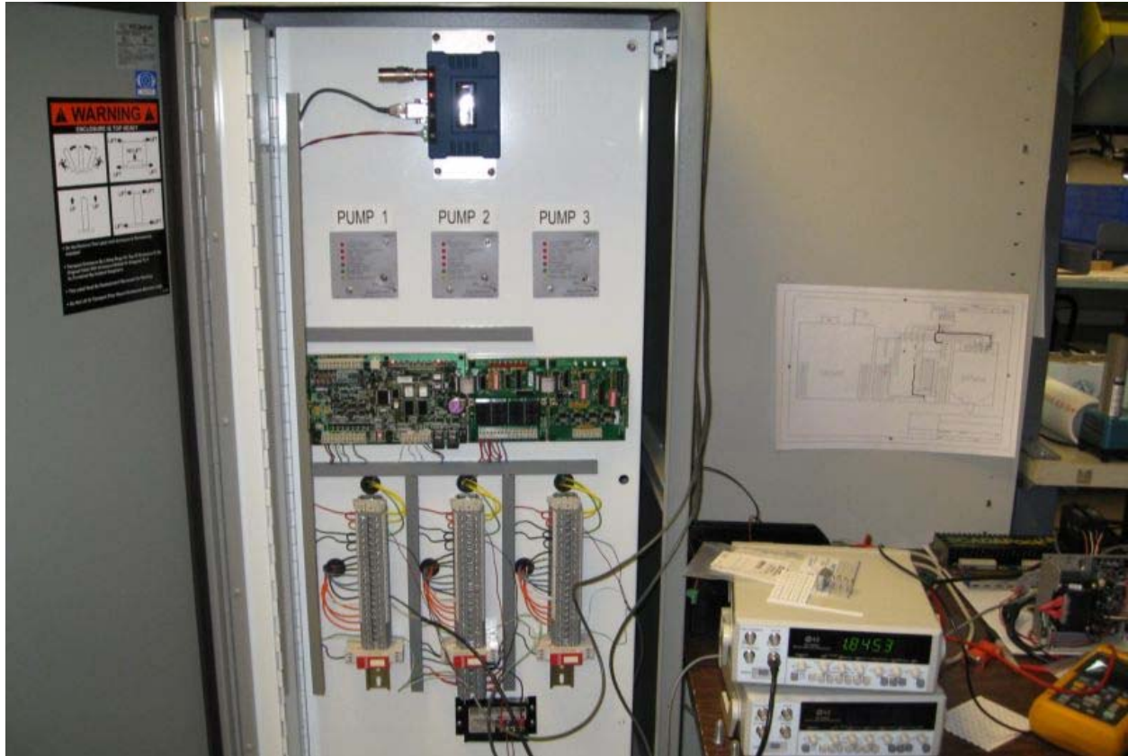
Figure 8 – Delta Lake Irrigation District – Variable Speed Controller
