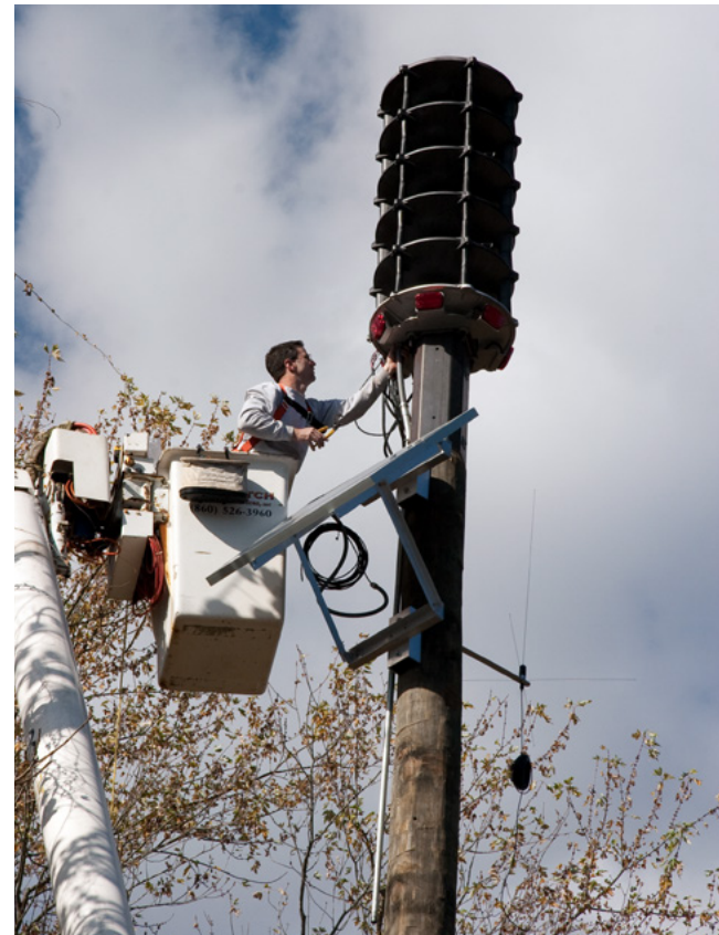
Whelen omni-directional WPS2906 siren being installed
