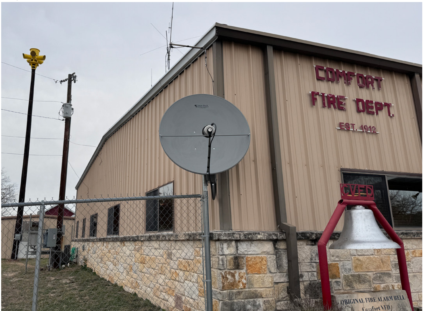
Sentry Siren omni-directional 14v siren installed at the Comfort, Texas fire department
