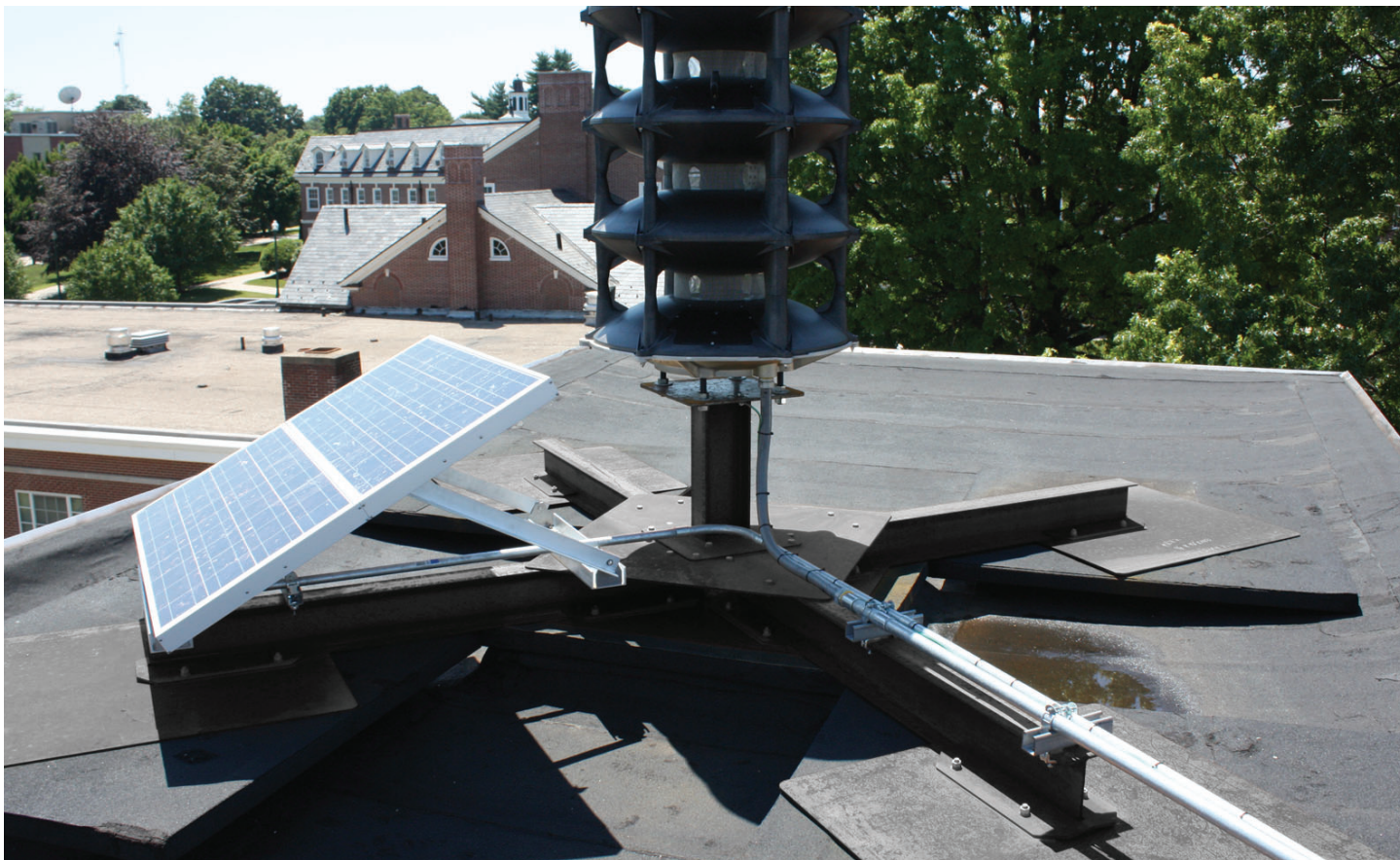
Whelan WPS-2903 siren mounted on a roof
