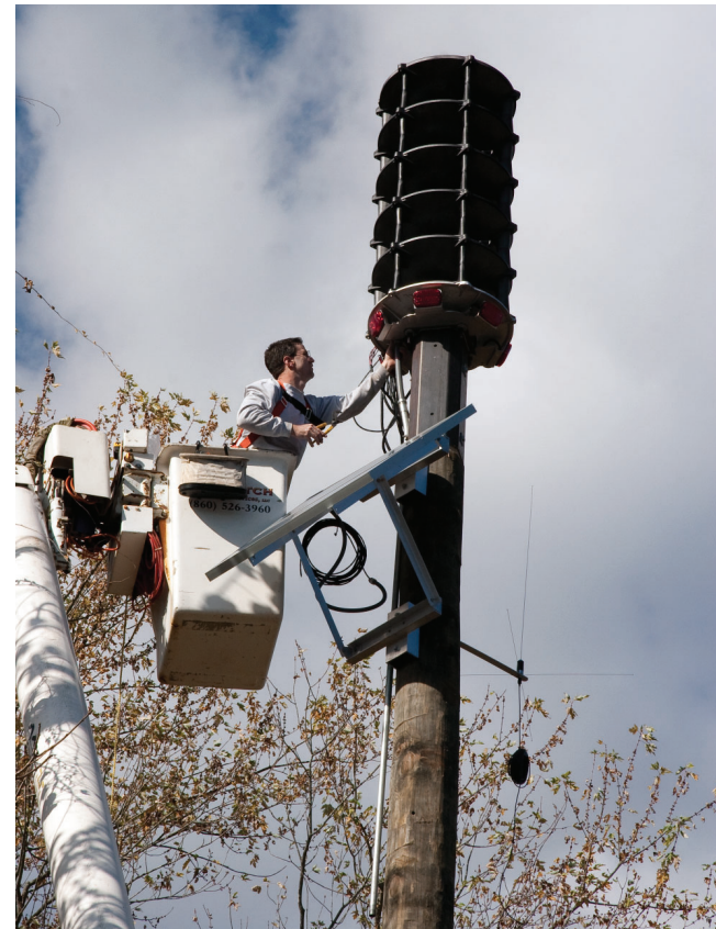
Whelen omni-directional WPS2906 siren being installed
