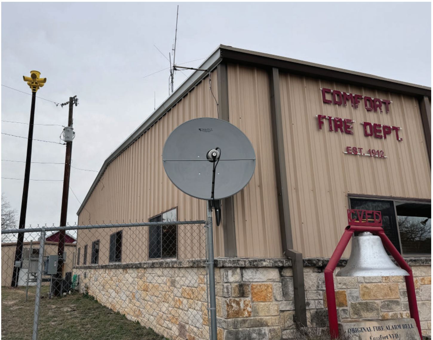
Sentry Siren omni-directional 14v siren installed at the Comfort, Texas fire department
