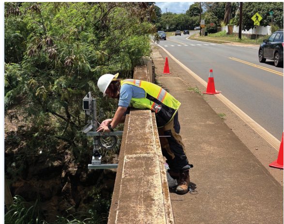
Installation of river gauge on a roadway
