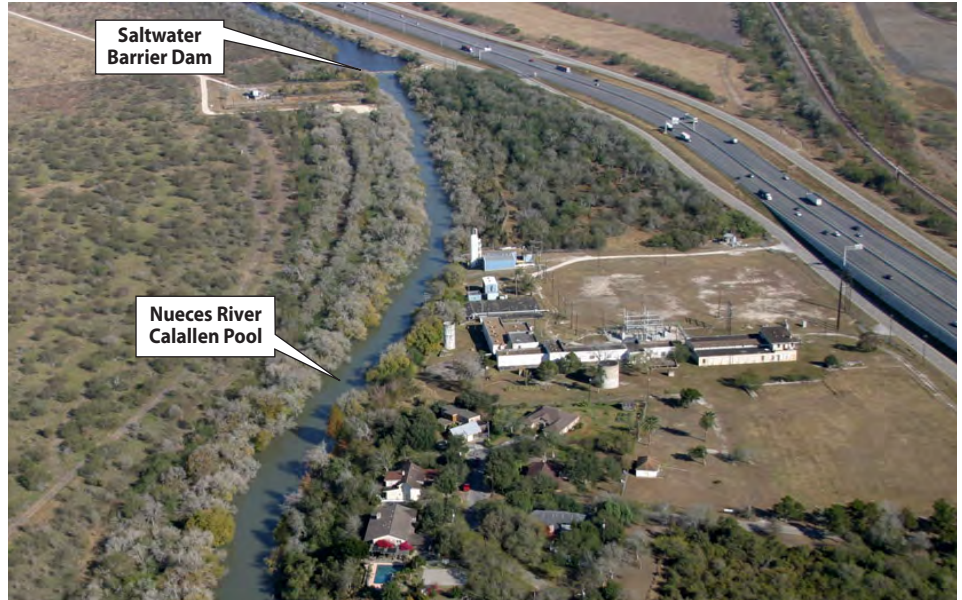
Five municipal and industrial pump stations withdraw water from the Nueces River pool behind the Calallen Saltwater Barrier Dam alongside Interstate 37.
