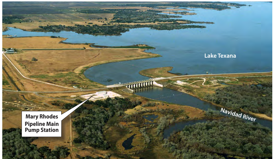
Palmetto Bend Dam creates the 11,000-acre Lake Texana in Jackson County. Lake water is delivered to Coastal Bend customers through the 101-mile long, 64-inch diameter Mary Rhodes Pipeline.
