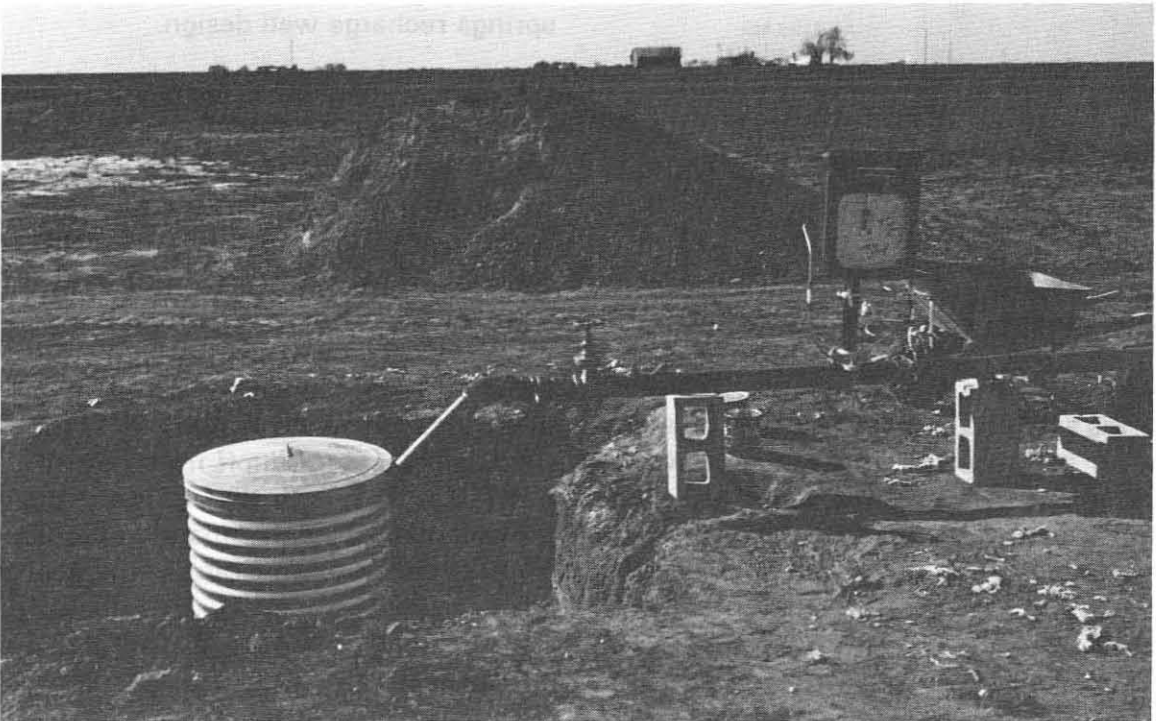
Figure 8-15.—Air Injection Hole With Pressure Recording Devices
