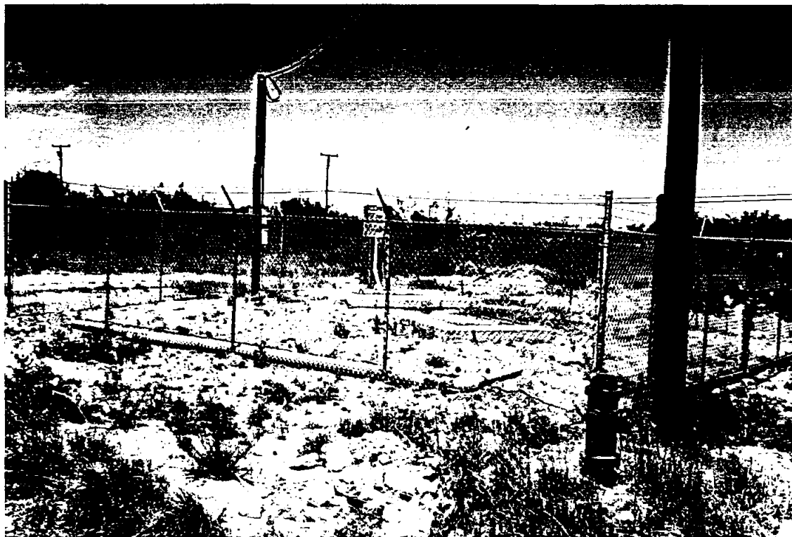
EAST U.S. HWY. 90 SEWAGE LIFT STATION 2 - SUBMERSIBLE-TYPE PUMPS
