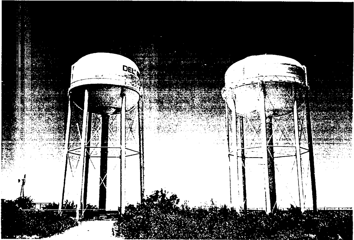
ELEVATED STORAGE NORTH OF AGARITA DRIVE 1 - 500,000 - GALLON (LEFT) 1 - 750,000 - GALLON (RIGHT)
