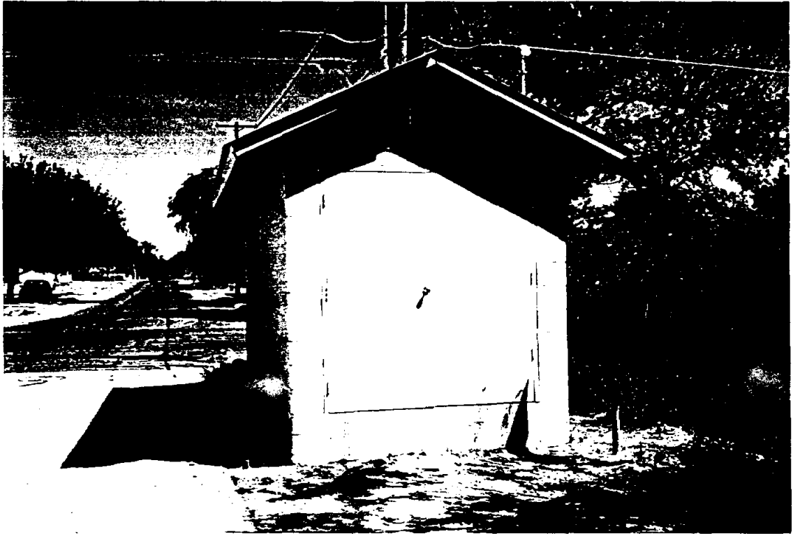
PIERCE AND HOLMIG STREETS SEWAGE LIFT STATION
