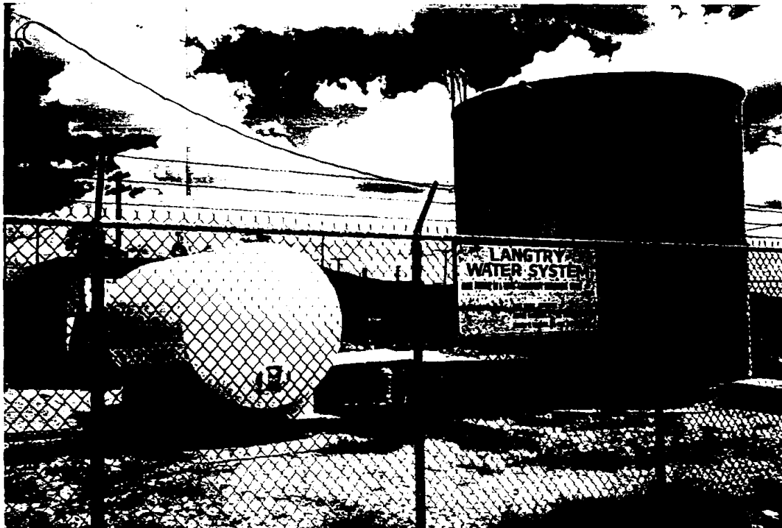
27,500 - GALLON GROUND STORAGE TANK (RIGHT) 2,500 - GALLON PRESSURE TANK
