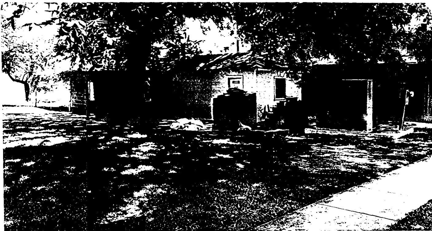
SAN FELIPE SPRINGS PUMPING STATION (EAST FACILITY)
