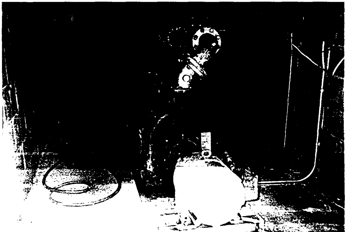
SINGLE SELF-PRIMING-TYPE PUMPING UNIT AT THE PIERCE / HOLMIG STATION
