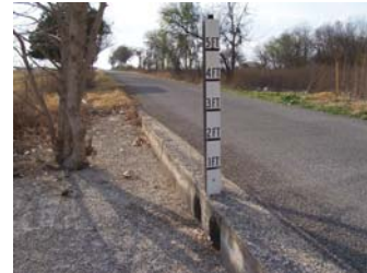
Figure 14: Low-water crossing at Haeckerville Road
