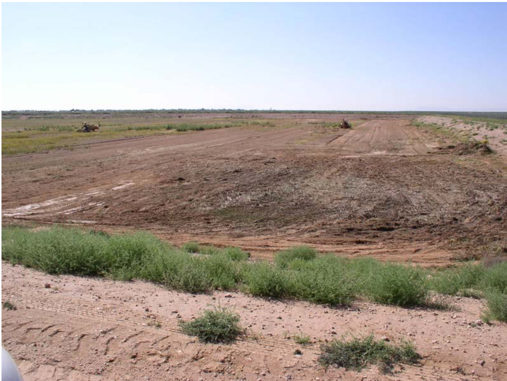
Figure 12-10. Horizon MUD south pond (not active) being scraped
