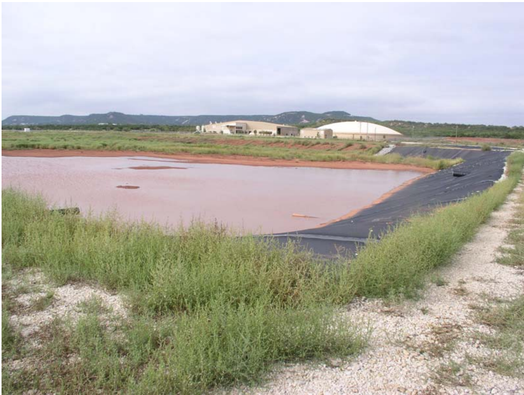
Figure 12-13. City of Abilene west pond showing the liners employed to control wave action
