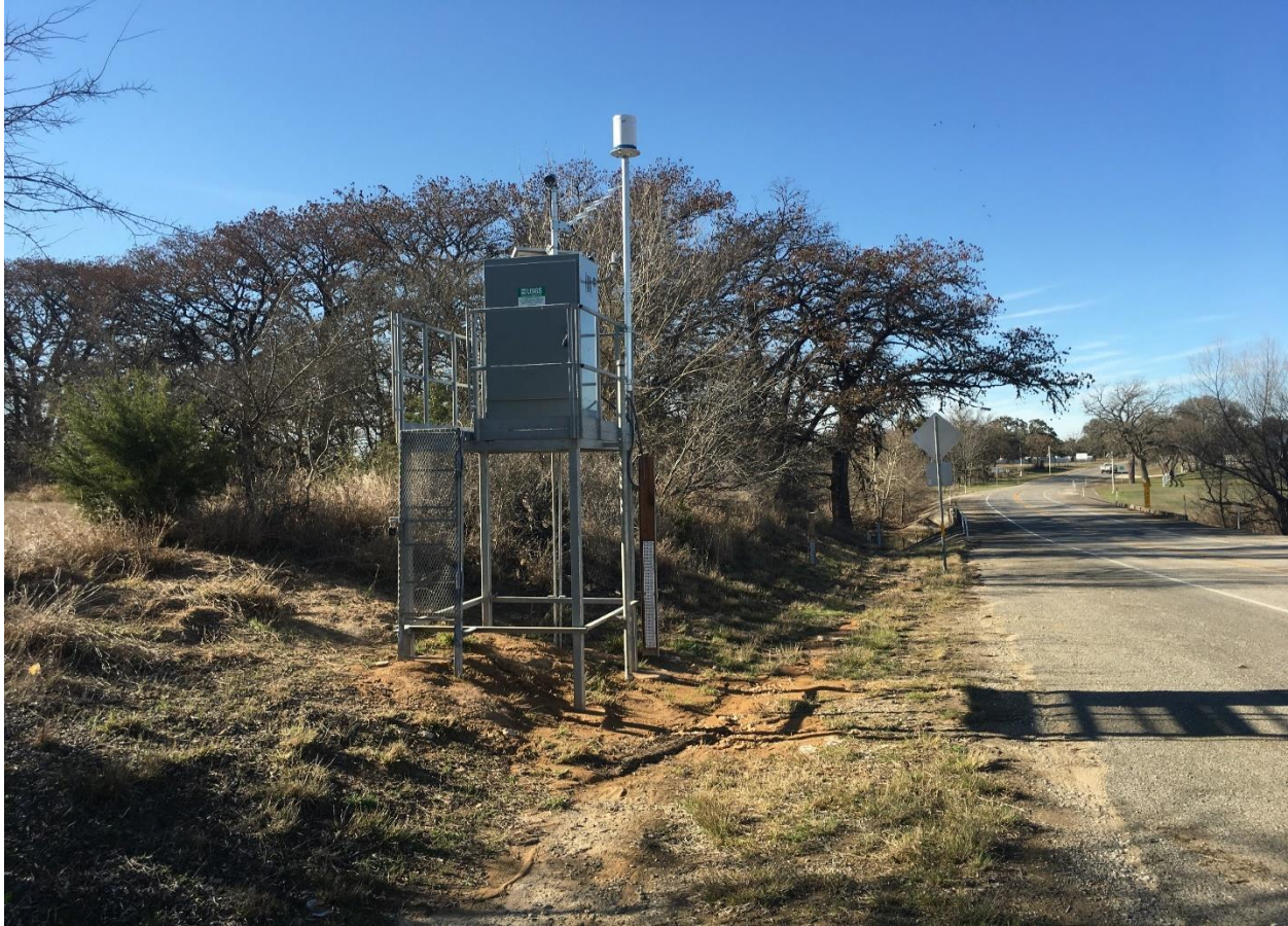
Figure 11-1, USGS Base Reference Stream Gage 08197970 at the Sabinal River Bridge at Utopia, Tx FM-1050 for the Sabinal River FEWS
