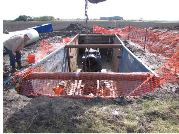
Preparing for dry bore.
