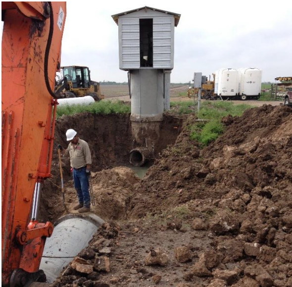
Tying into Pumping Station 55.
