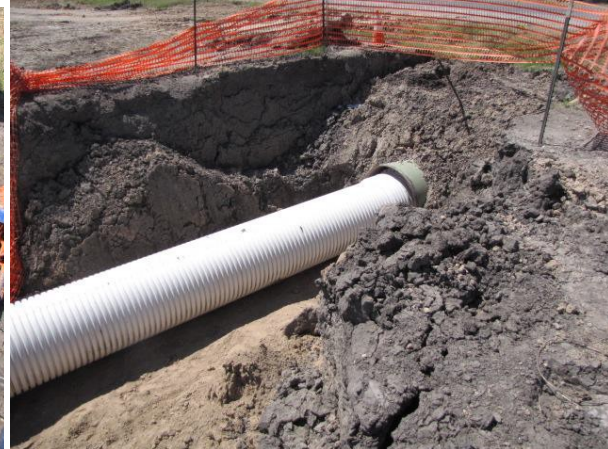
Completed dry bore with 30-inch pipe installed
