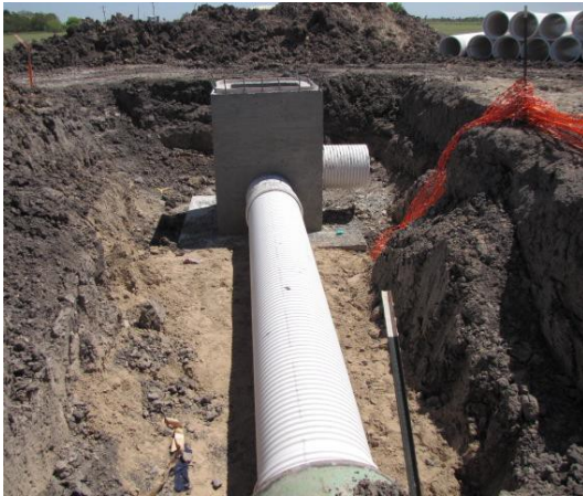
30-inch pipeline going south.
