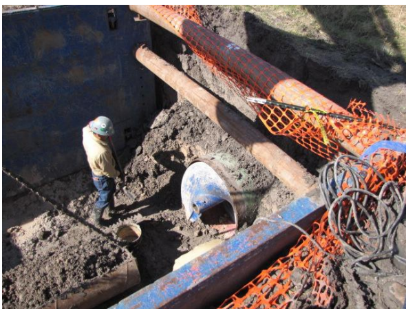
Dry bore in progress.
