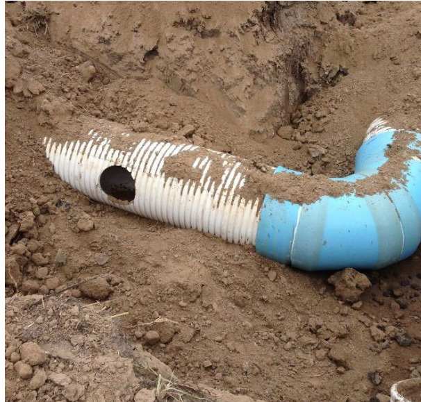
Hole for a turnout.
