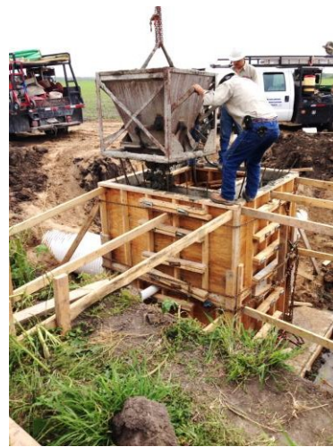
Pouring a junction box.
