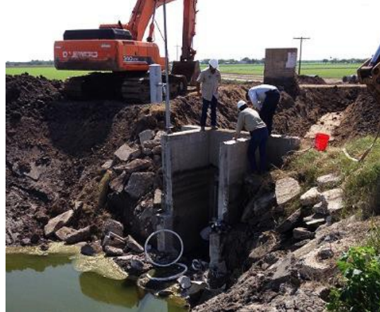
The images above show the outlet control structure from McLeod Hood Reservoir. The District replaced the gate and cut the concrete box down to allow for more flow from the reservoir.
