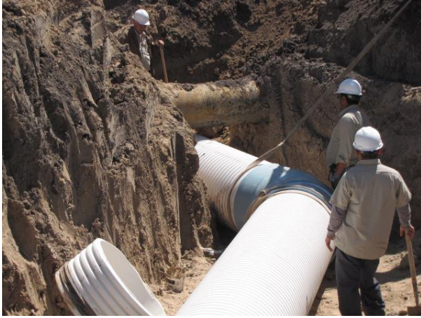
Working around a municipal water line.
