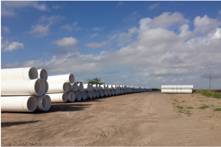
Pipe staging area.
