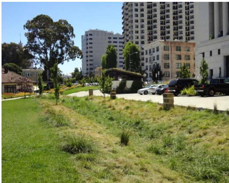
Figure 9: Vegetated Swale at Lake Merritt, Oakland, California Source: Watearth, Inc.
