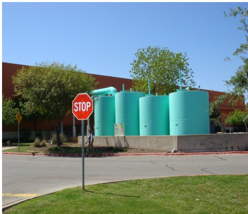
Figure 11: 28,000-Gallon Cisterns for Rainwater Harvesting on Brodie Lane, Austin, Texas Source: Watearth, Inc.
