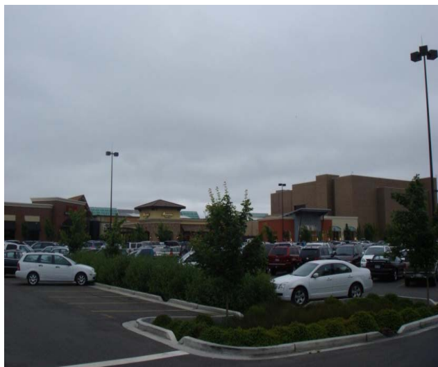
Figure 7: Commercial Parking Lot Application of Bioretention, Northgate Mall, Seattle
