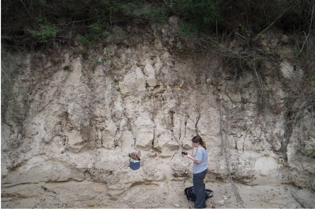
Figure B5: Tributary to Big Gulch Bayou, Failing Channel Banks
