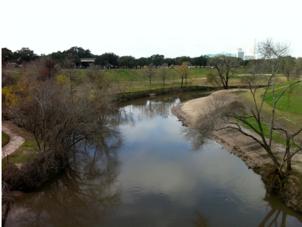
Figure B8: Buffalo Bayou at Sabine Street – Just After Construction, Prior to Planting
