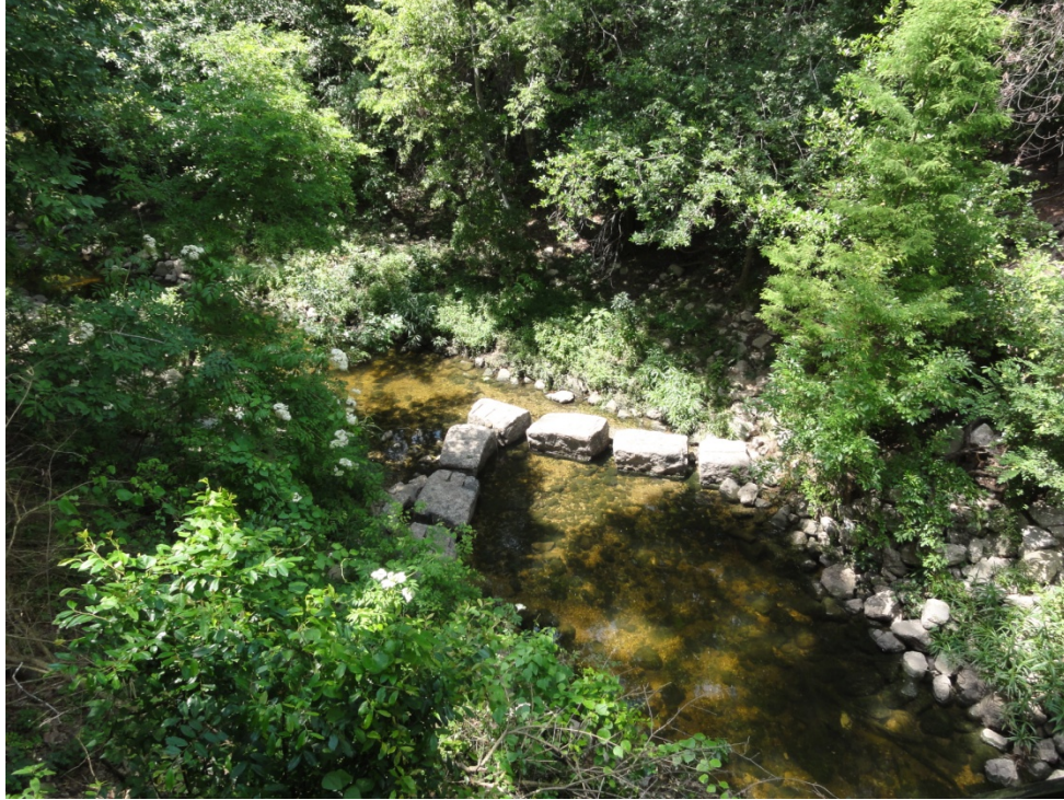
Figure B13: Rummel Creek after stabilization (2012)
