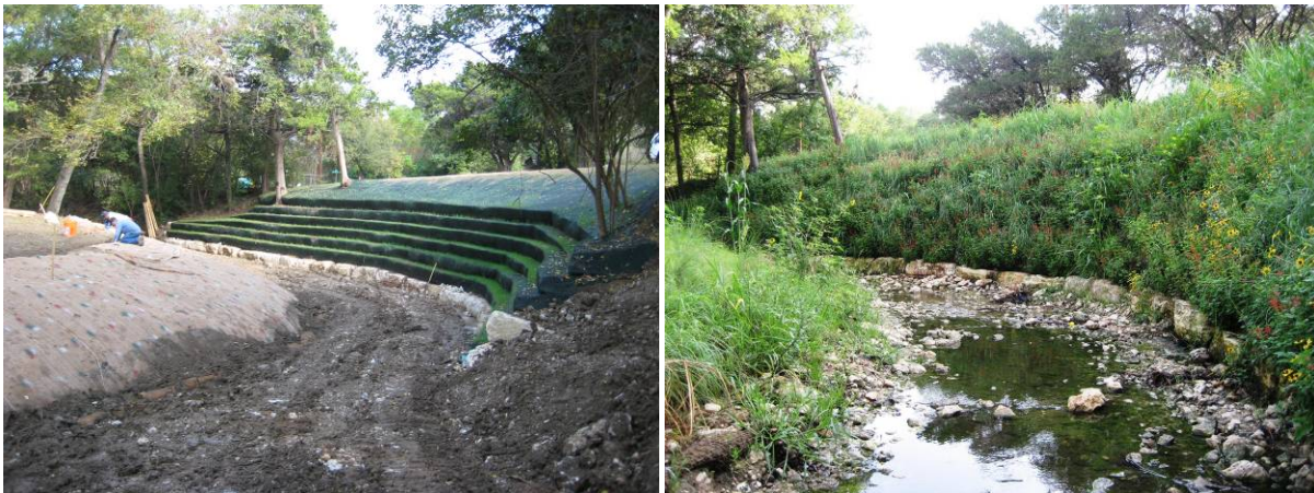
Figure 15: City of Austin Typical Stacked Boulder Wall Installation
