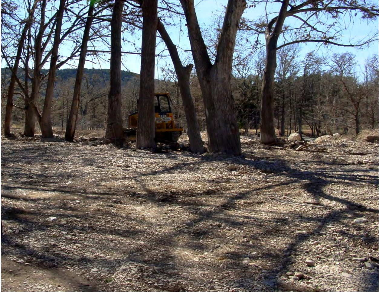
Figure 7.19. Disturbance with heavy equipment along the banks for floodplain will often result in large additions of sediment to the channel, which disrupts the balance. Photo courtesy of Sky Lewey, Nueces River Authority.
