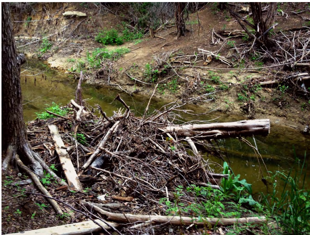
Figure 6.6: A recently deposited debris pile partially obstructing streamflow along a headwater stream. The stream is in a semi-urban setting, and debris includes both human-contributed and natural debris. (photo by J. Duke)
