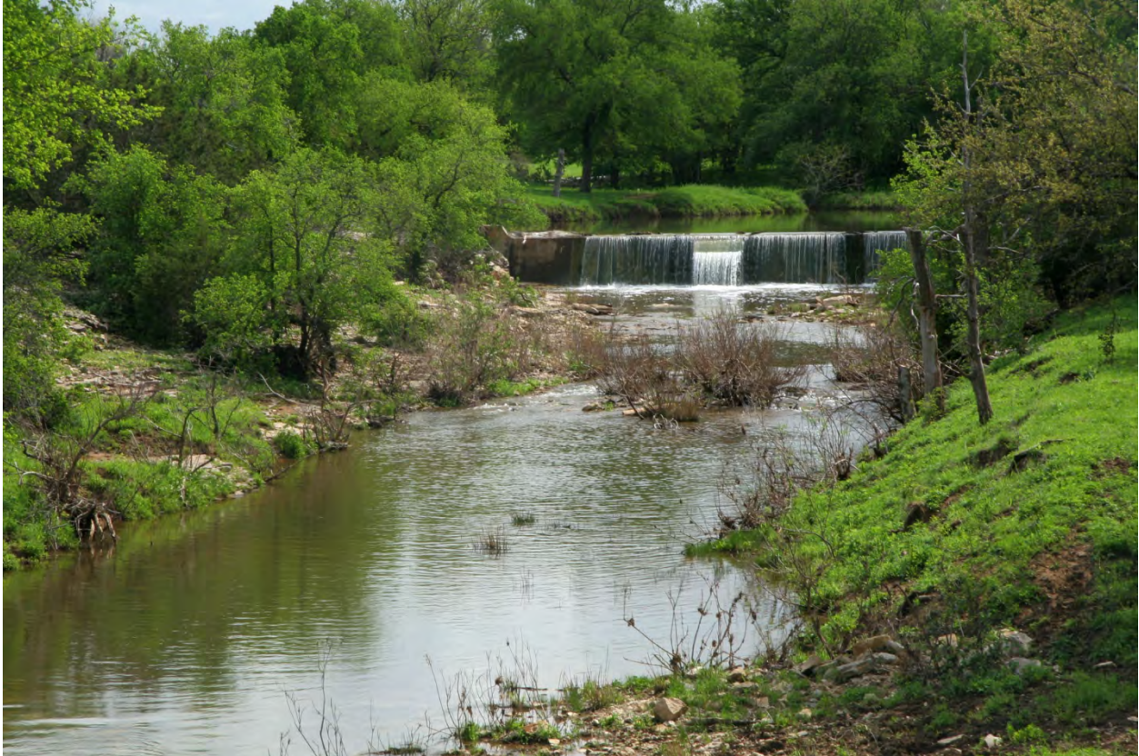
Figure 7.26. Thousands of low head concrete dams have been built on Texas creeks. These dams disrupt the natural movement of sediment that is needed downstream to build point bars and sinuosity. Erosion is often accelerated below the dams, creating additional problems. Some landowners are now considering the removal of these dams. Photo courtesy of Ricky Linex, NRCS.
