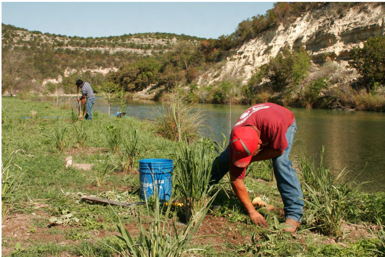
Figure 7.29. Various artificial re-vegetation techniques are used to jump-start the development of riparian vegetation. Re-seeding and transplanting have been successfully used in riparian restoration projects.
