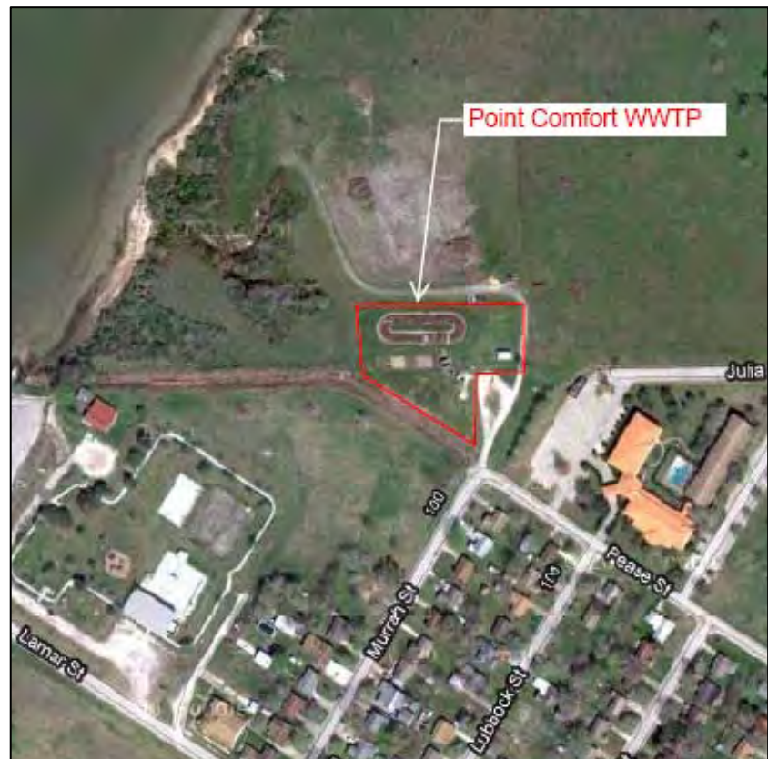
Figure 3-1 City of Point Comfort WWTP
