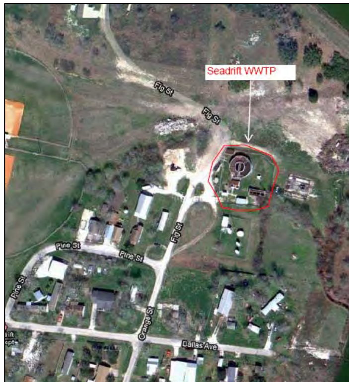
Figure 3-3 City of Seadrift WWTP
