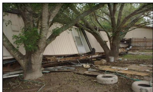
Flood Damage in Timber Creek, November 2001
