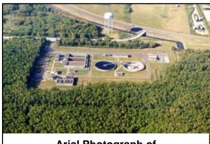
Arial Photograph of Groves WWTP
