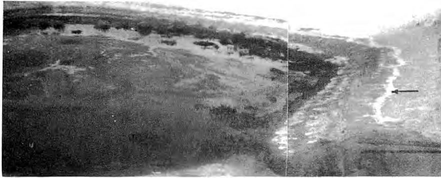
Figure 11.--Unlined surface disposal pit on Carl Lockhart lease, NW $\frac{1}{4}$  Section 34, Block 32, T-3-N, T & P RR Survey, Howard County. Pit is constructed in permeable conglomerate shown in Figure 4 and 5. Former level of brine is indicated by salt precipitate (arrow). Waste crude oil and tank bottom residue remain in pit. View is northeast. Picture taken 4-22-64.
