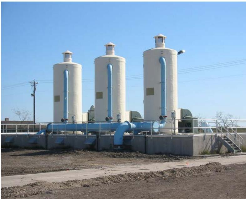
**Figure 1 - Finished Water Pump Station and Degasifier**
