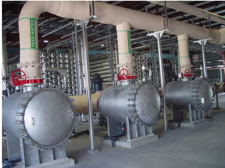
**Figure 8 - Cartridge Filtration Pretreatment**
