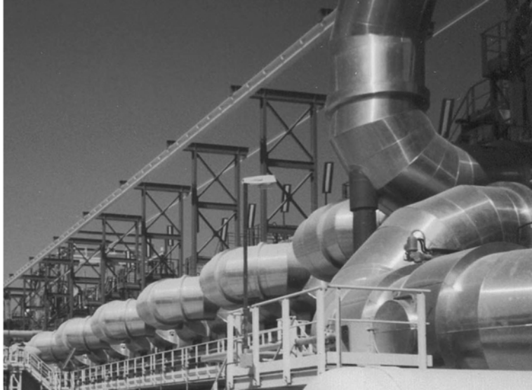
Figure 2 Multistage flash distillation in Abu Dhabi Emirate
