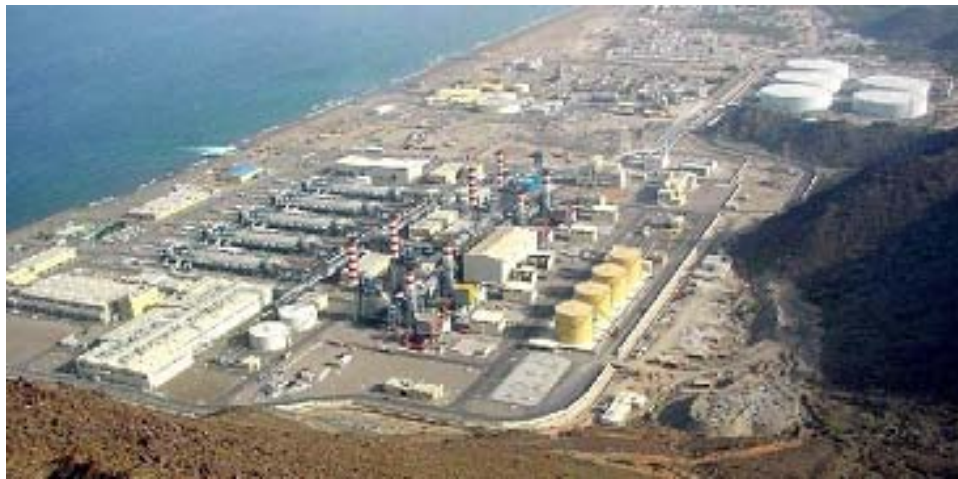
Figure 9 - World's largest hybrid - 78 mgd multi-stage flow and 45 mgd seawater reverse-osmosis [Photo courtesy of Doosan]
