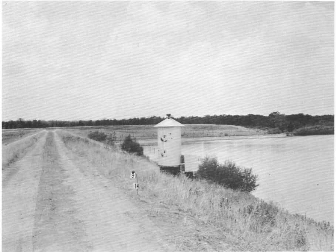
Figure 4.—Typical Gage Installation at a Floodwater-Retarding Reservoir
