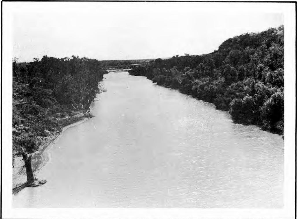
Looking downstream from the old silt sampling station. The river flow was 184 acre feet per day and the silt content amounted to 8 tons for the day. The water was practically clear. A small gravel dam was made by the State Highway Department, as may be seen in picture, to secure gravel for new bridge being constructed upstream. The dam backed the water up beyond the station.
