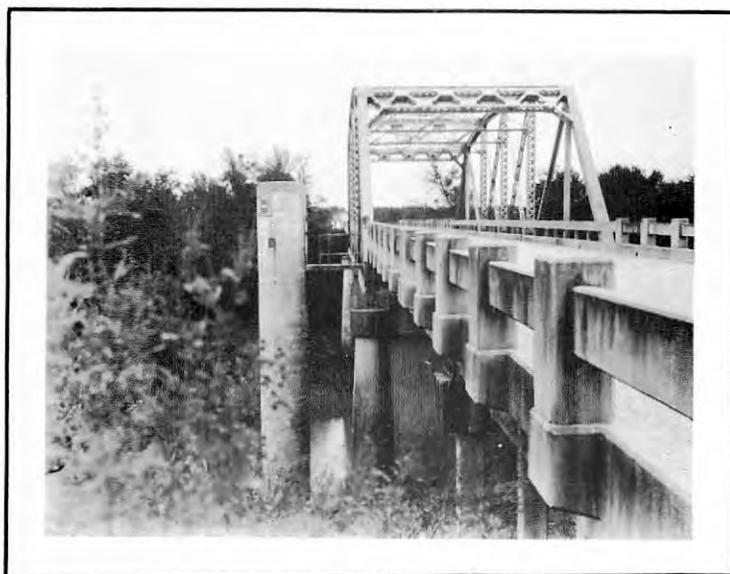
Bridge on U. S. Highway 59 between Goliad and Berclair where water samples are obtained for silt determinations. The samples are taken near U.S.G.S. gaging station which is located on the upstream side of the bridge.
