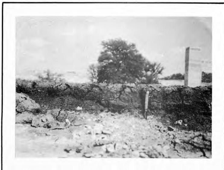
The depth of sediment deposited in front of this dam from one flood is approximately 4 to 5 inches as indicated by size of pocket knife. The silt contains little moisture and is well compacted.
