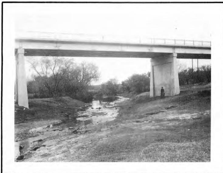
The silt sampling station is located at a bridge on U.S. Highway 81 near Cotulla. The Nueces River at this station usually has a very small flow and small amount of silt for the greater part of the year. The USGS wire gage may be seen attached to the bridge railing. Looking upstream.
