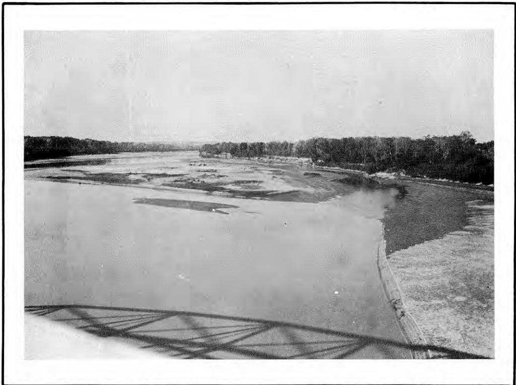
Looking upstream from silt sampling station. The stream channel is wide and sandy. There is considerable shifting of the main stream through the sandy channel. The Denison Dam is being constructed several miles upstream and at horizon in center of picture.
