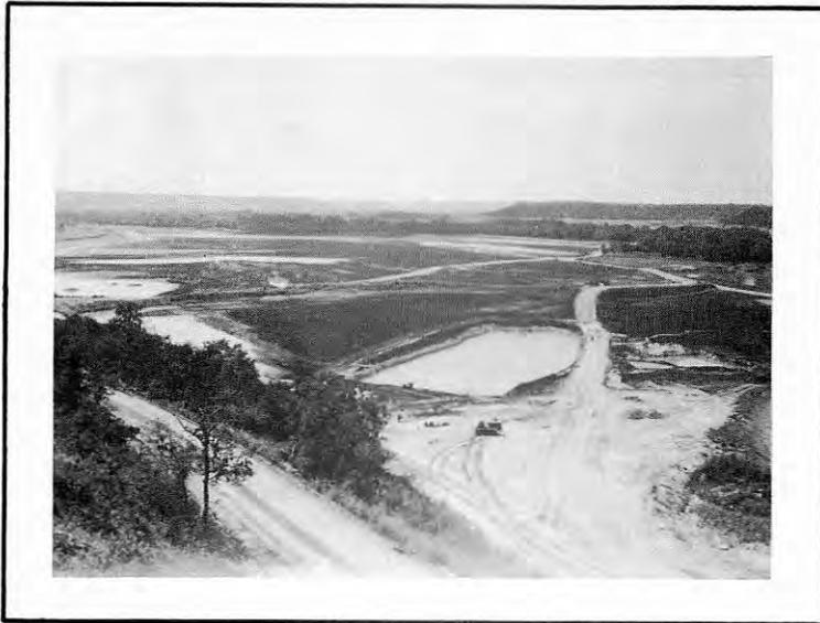
Sedimentation of a lake in Texas before a dam has been completed. The original top soil of the lake bed has been removed (down to white material) and used for construction of this particular dam. The black colored material is sediment deposited in front of the dam from one flood.
