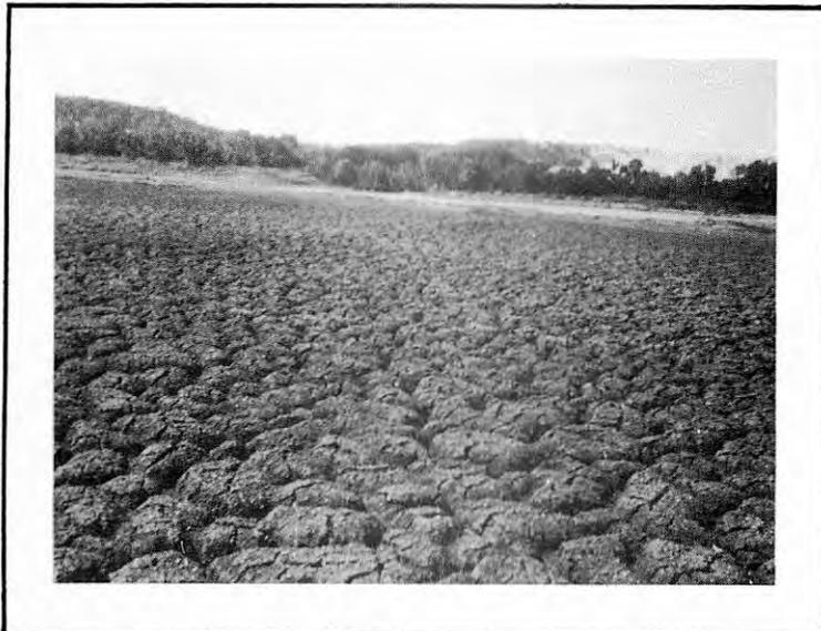
A close-up view of sediment deposited in front of one of Texas's dams as result of one flood. This sediment will remain behind dam unless removed by artificial means. The original storage capacity has been decreased by the sediment.
