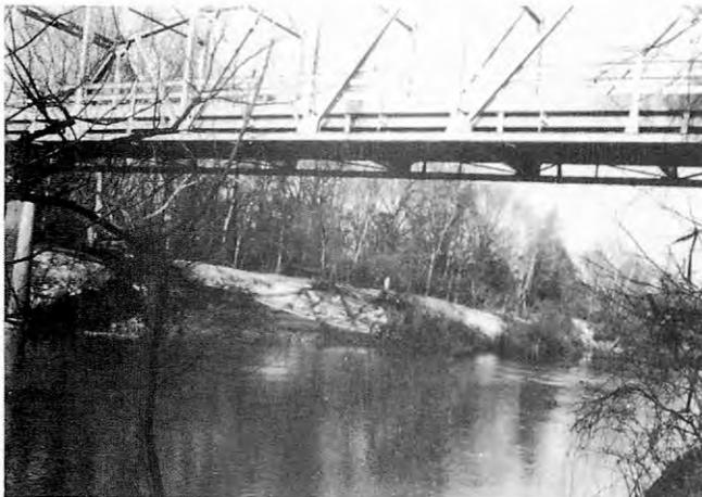
(above) Looking downstream from silt sampling station. The left fork is the location of several USGS staff gages for measuring heights of various stream flows. The regular stream channel is about 200 feet wide and rather deep. The discharge of the river on day picture was made was 12,575 acre feet and the silt load 2,396 tons or 1.6 acre feet.
