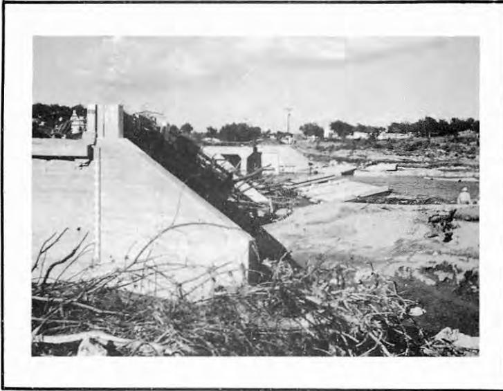
Bridge at silt sampling station on US-Highway 281 after September 10 and 11, 1952 flood. During the two-day flood, 360,000 acre feet of water washed away the bridge and silt station. This flood contained approximately 13,000,000 tons of silt or about 8,300 acre feet. The drainage area above the station is 947 square miles. The amount of silt per square mile of watershed area was nearly 9 acre feet which is the largest amount of silt for any watershed studied in Texas.
