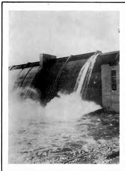
Silt sampling station at Possum Kingdom Dam. The water samples are obtained in the tailrace below power house at right in picture, or during floods, at both the usual location and at spillway of dam. During one year as much as 16 percent of the silt entering Possum Kingdom Lake by-passed the dam. The average amount by-passing the dam is 3 percent.
