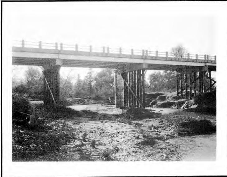
Bridge on U. S. Highway 79, between Marquez and Easterly, where water samples are obtained. The U.S.G.S. stream gaging station (concrete pipe) is located downstream and at center bent of wooden bridge piling. The small river discharge is characteristic of this stream most of the year as well as the silt content of the water.
