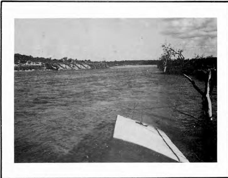
Looking downstream from the bridge and silt station that were destroyed by the 2-day September flood. The concrete floor of steel bridge is noticeable on river bank and remainder of USGS concrete tower gaging station is seen at bottom of picture. A week after the flood the river was discharging 1908 acre feet per day and this flow is shown in the picture.
