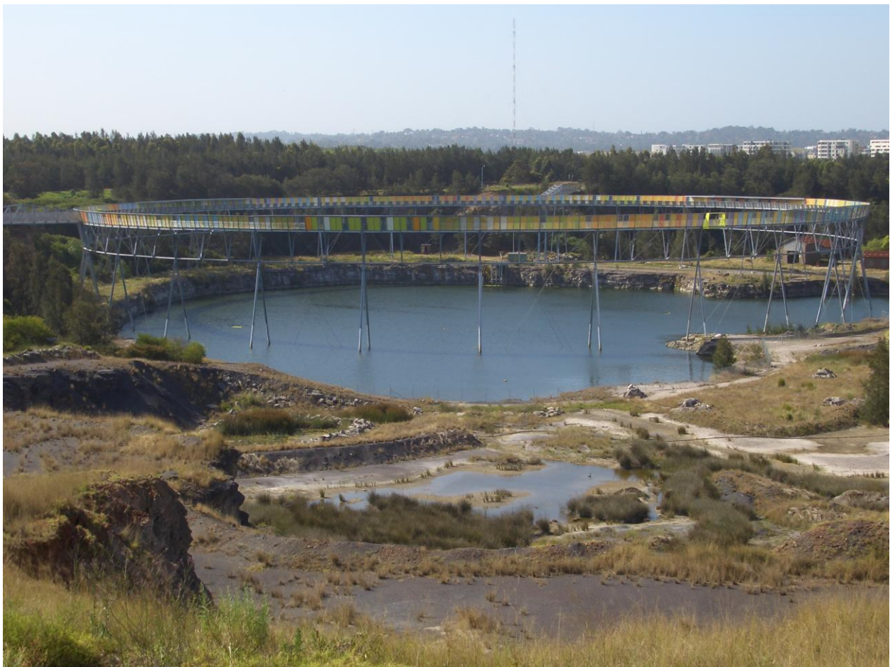
Figure 8-8: Brick Pit Storage at Homebush Bay
