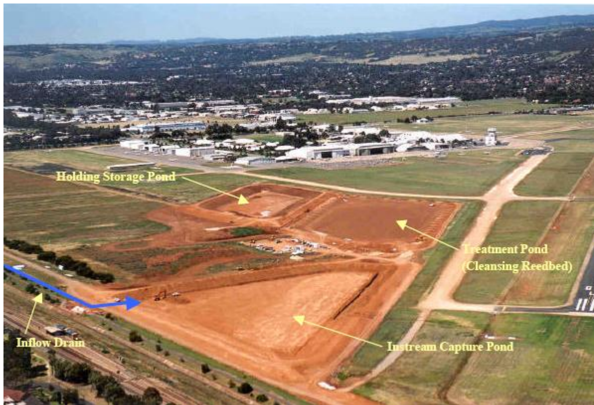
Figure 8-6: Construction of the Parafield Stormwater Harvesting Facility
