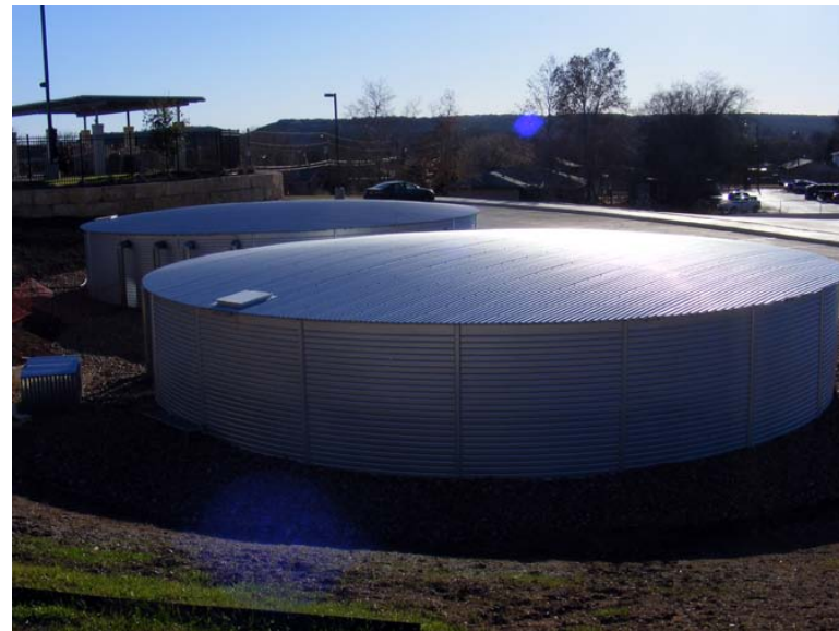
Galvanized metal tank with food-grade liner, Salvation Army Recreation Center, Kerrville
