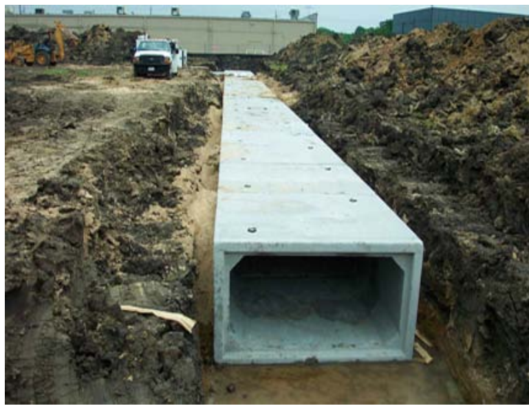
Medical Center, Webster (approximately 175,000 gallon capacity, concrete culverts under parking lot, green roof, irrigation and indoor toilet flushing use)
