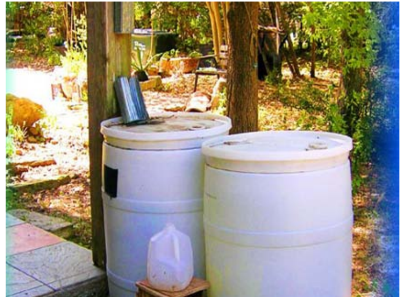
PermaCulture Center, Sunset Valley (approximately 1,750 gallon capacity, rain barrels, potable and non-potable use)
