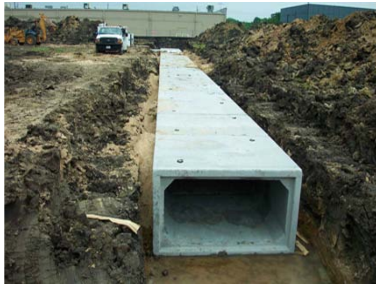
Concrete culverts (Medical Center, Webster)
