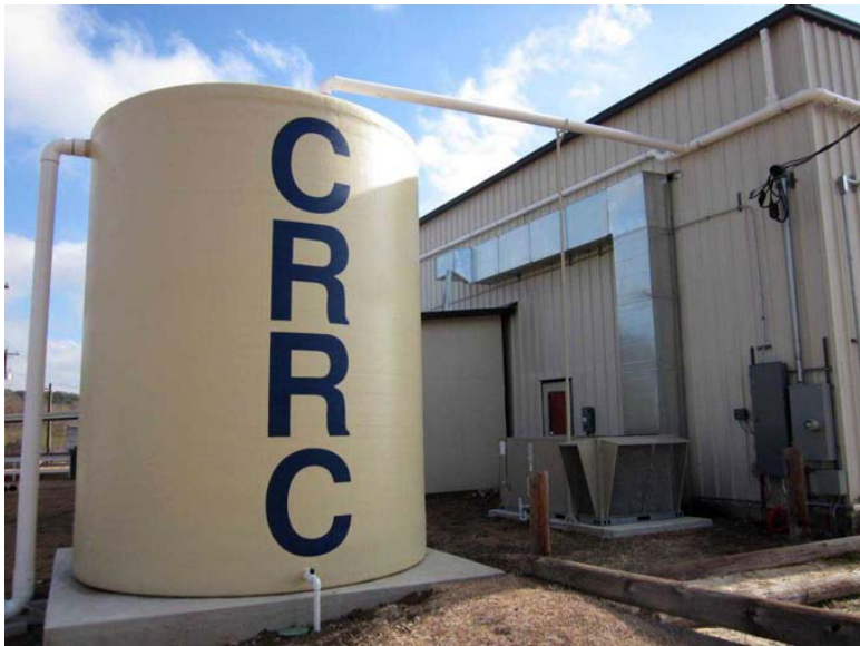
Community Resource and Recreation Center, Canyon Lake (12,500 gallon capacity, installed to control stormwater flow)
