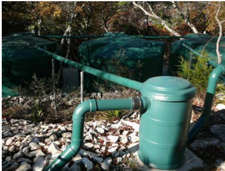
First-flush washer with sock filter, Kight residence, Boerne
