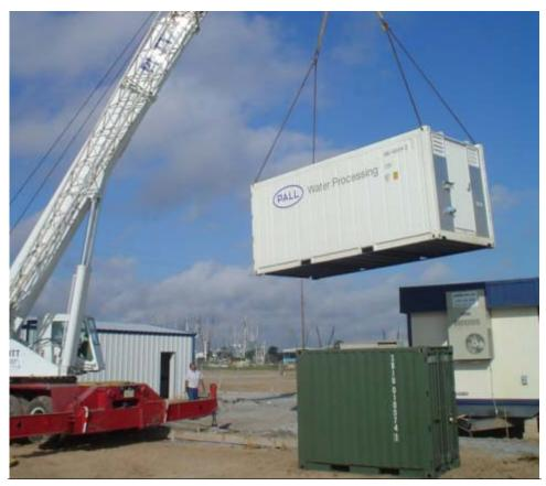
Figure 2-9: Photograph showing the placement of the Pall pretreatment unit.
