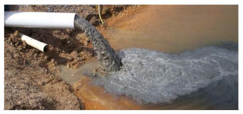
Figure 4-1: Photograph of discharge into the lagoon from flushing the raw water manifold. Flushing was periodically required to eliminate the buildup of sediment and other debris in the manifold line.
