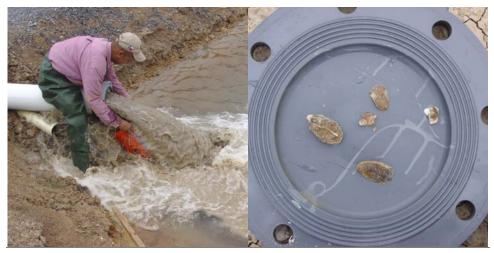
Figure 4-2: Photograph of sampling for shell fragments and other large debris being discharged during flushing of the raw water manifold (left) and examples of some shell materials recovered (right).
