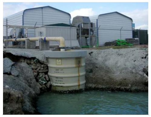
Figure 2-5: Photograph of the raw water intake structure.
