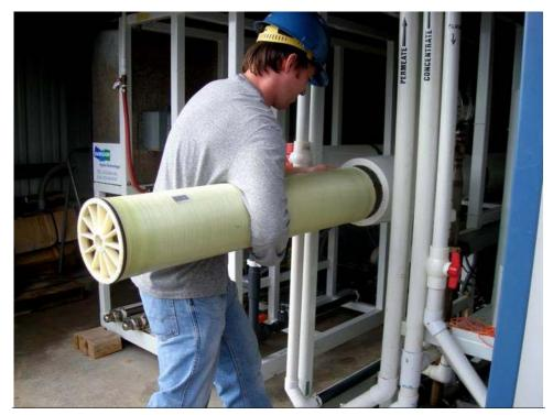
Figure 2-10: Photograph showing the loading of an RO element into the pressure vessel.
