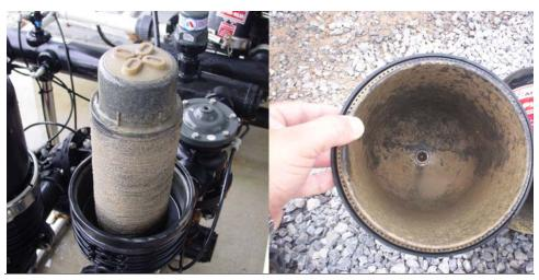
Figure 3-13: Photograph of sediment buildup in the discs (left) and hood (right) of one of the GE Zenon Arkal units.
