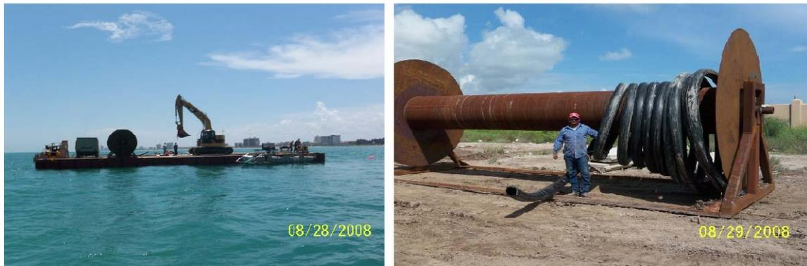
**Figure 9 - Barge installing open ocean intake off South Padre Island and transmission pipe**
