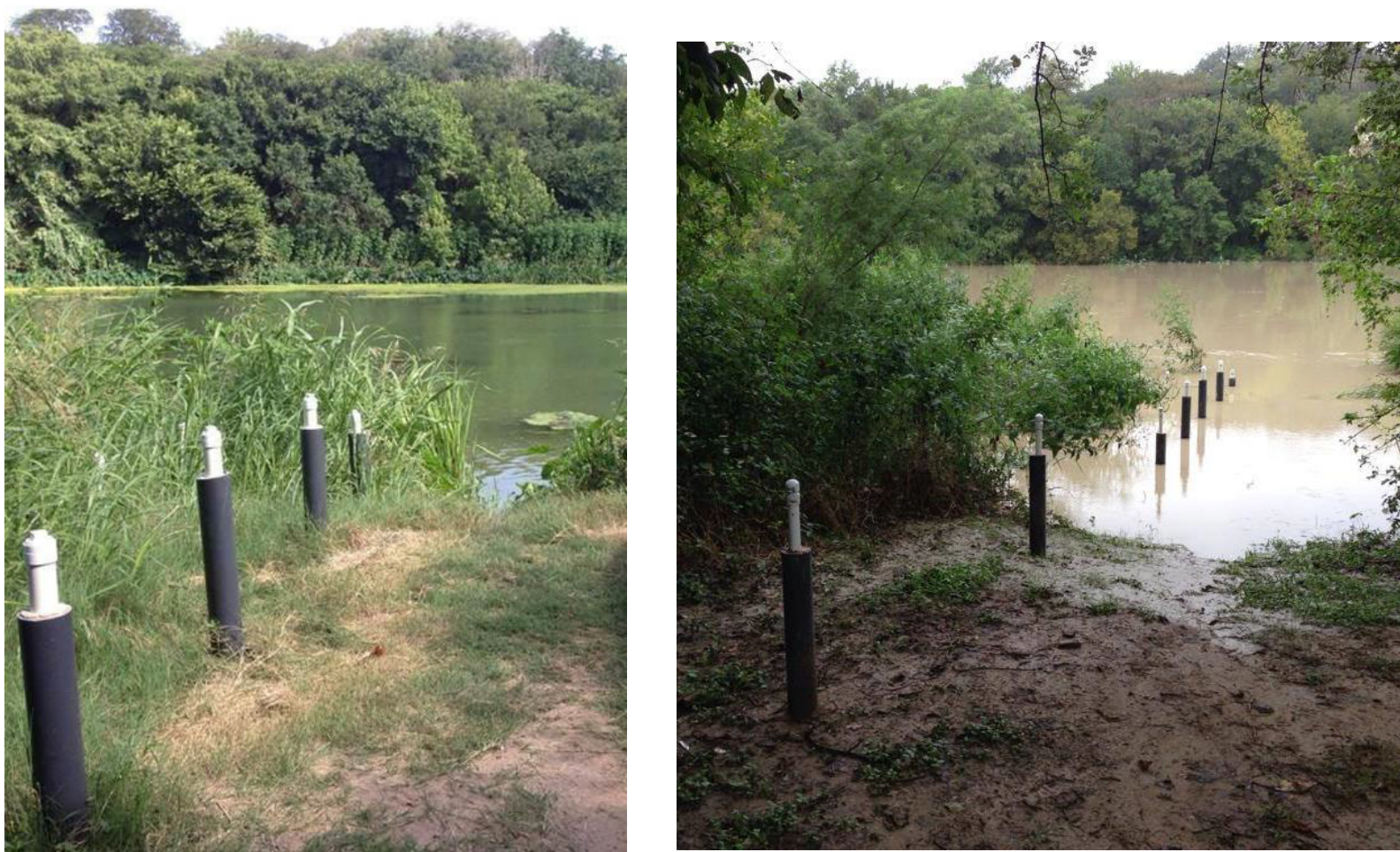
Figure 7-2. Network of monitoring well installed in the Colorado River alluvium at Hornsby Bend using a Geoprobe System under flow conditions (A) and after a 10,000-cubic-foot-per-second storm event (B) (from Barrera, 2015).
