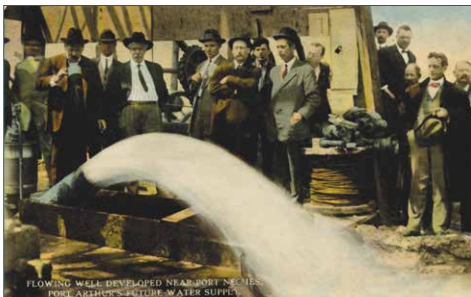
FIGURE 9. Flowing artesian well developed for the Port Arthur, Texas, water supply (circa 1910).
