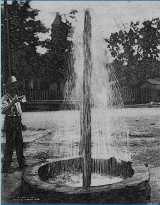
FIGURE 24. A flowing artesian well in Hallettsville, Texas. Source: Fey and Braunig, Artesian Well, Photograph, n.d.; digital images, ( texashistory.unt.edu/ark:/67531/metaph128796/m1/1/ ), University of North Texas Libraries, The Portal to Texas History, texashistory.unt.edu ; crediting Friench Simpson Memorial Library, Hallettsville, Texas.
