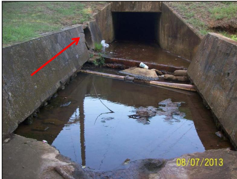
**Photo 2 – 24" RCP outfall of North Subsystem A**
