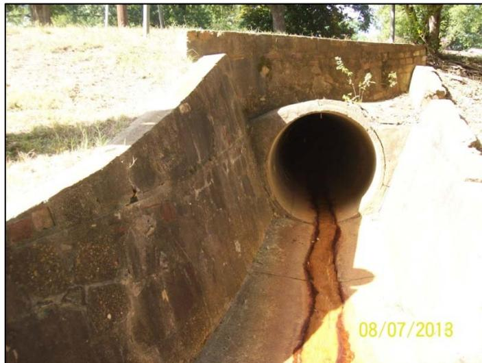
**Photo 3 – South System 48" RCP outfall to concrete lined channel north of E. Kay Street**
