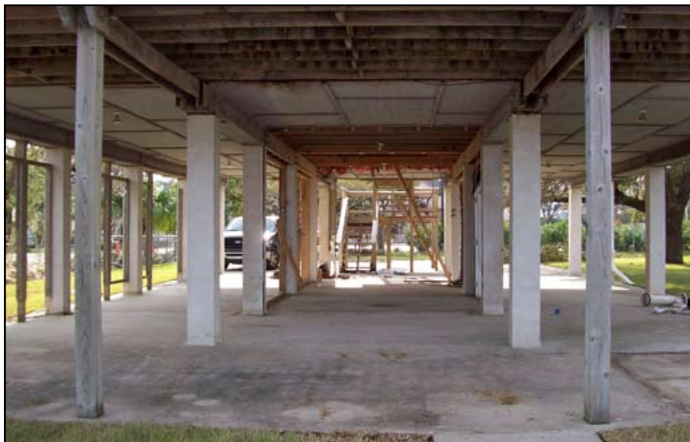
Breakaway walls gone with the storm.
