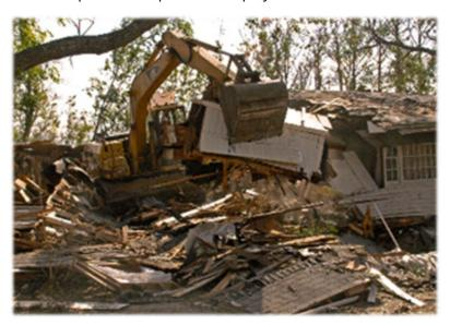
Figure 1. A photo of a large excavator demolishing a house.
