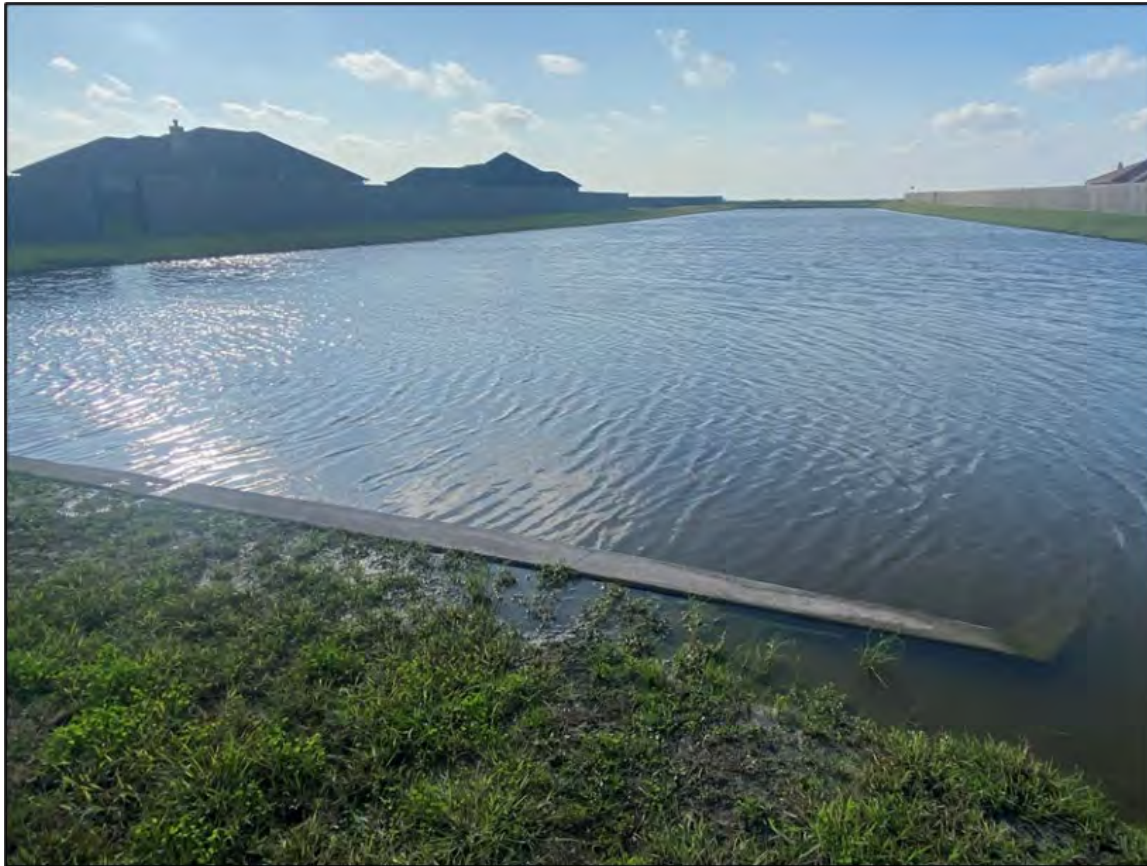
Figure 1.5 Nottingham Acres Subdivision Pond with Water Above the Headwall
