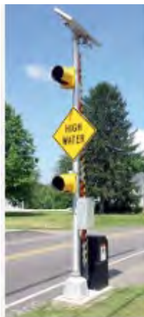
Figure 7-21. Example of a flood detection warning system with gate closure.
