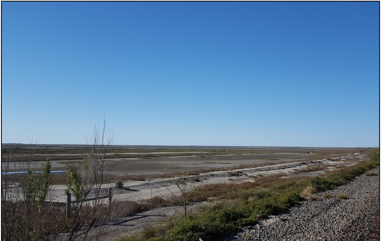
Figure 8. Allison Wastewater Treatment Plant Discharge Demonstration Site (January 30, 2017).
