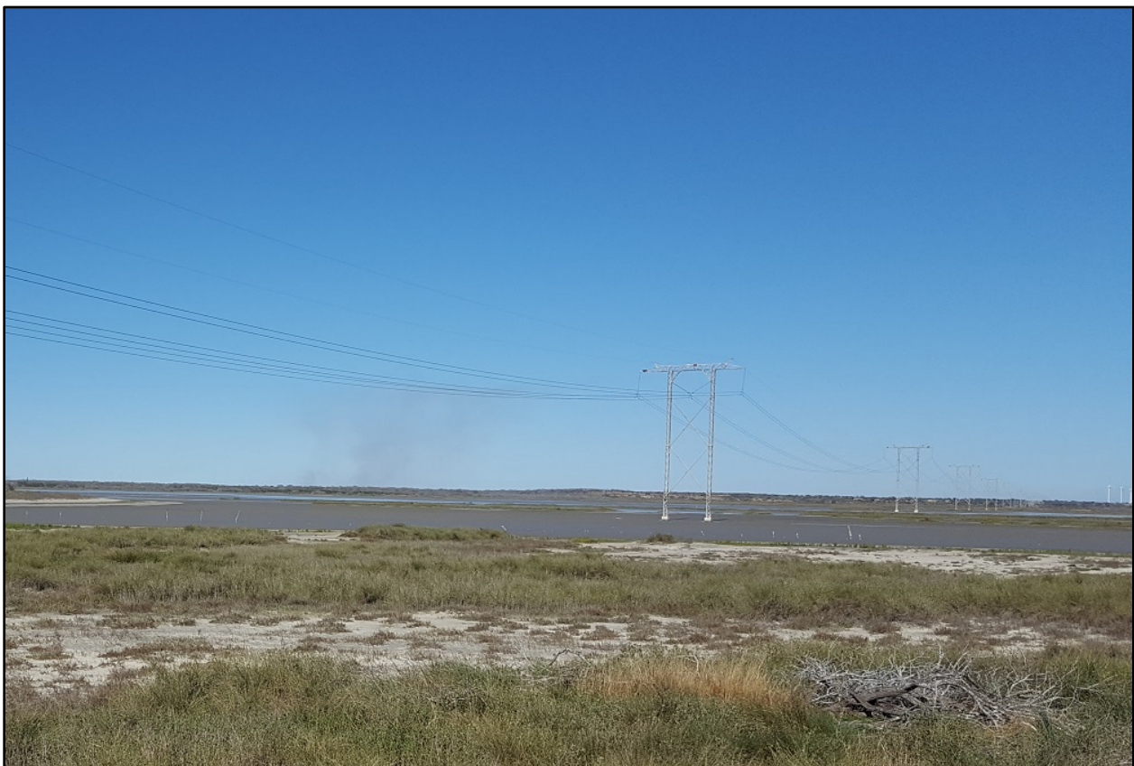
Figure 19. Middle Rincon Bayou. View from south shore towards north. (Photo taken January 30, 2017).
