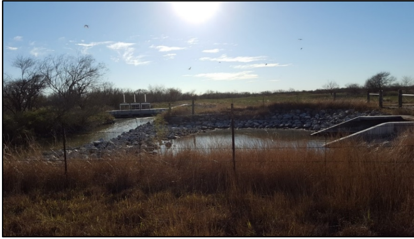
Figure 2. Rincon Bayou Diversion. View towards upstream with discharge point on the right and water control structure upstream. January 30, 2017.
