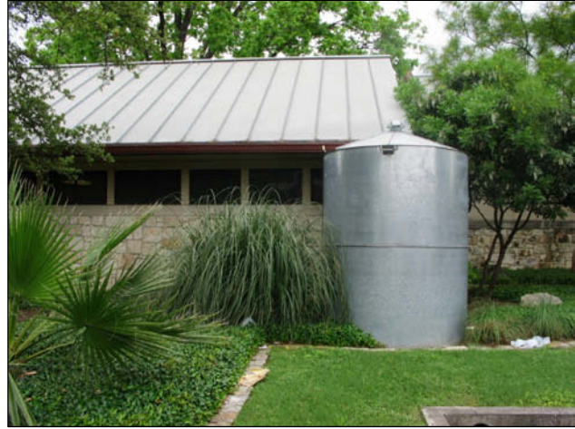
A 2,000-gallon, ranch-style metal cistern is one of two tanks that capture rainwater for landscaping at the Edwards Aquifer Authority building. (Photo courtesy: Lara Stuart)
